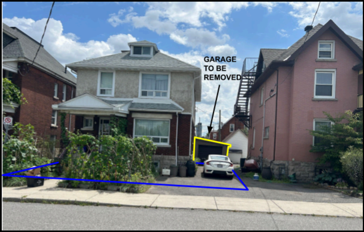
Image from Oak St looking south towards the subject property showing the property's boundary.
