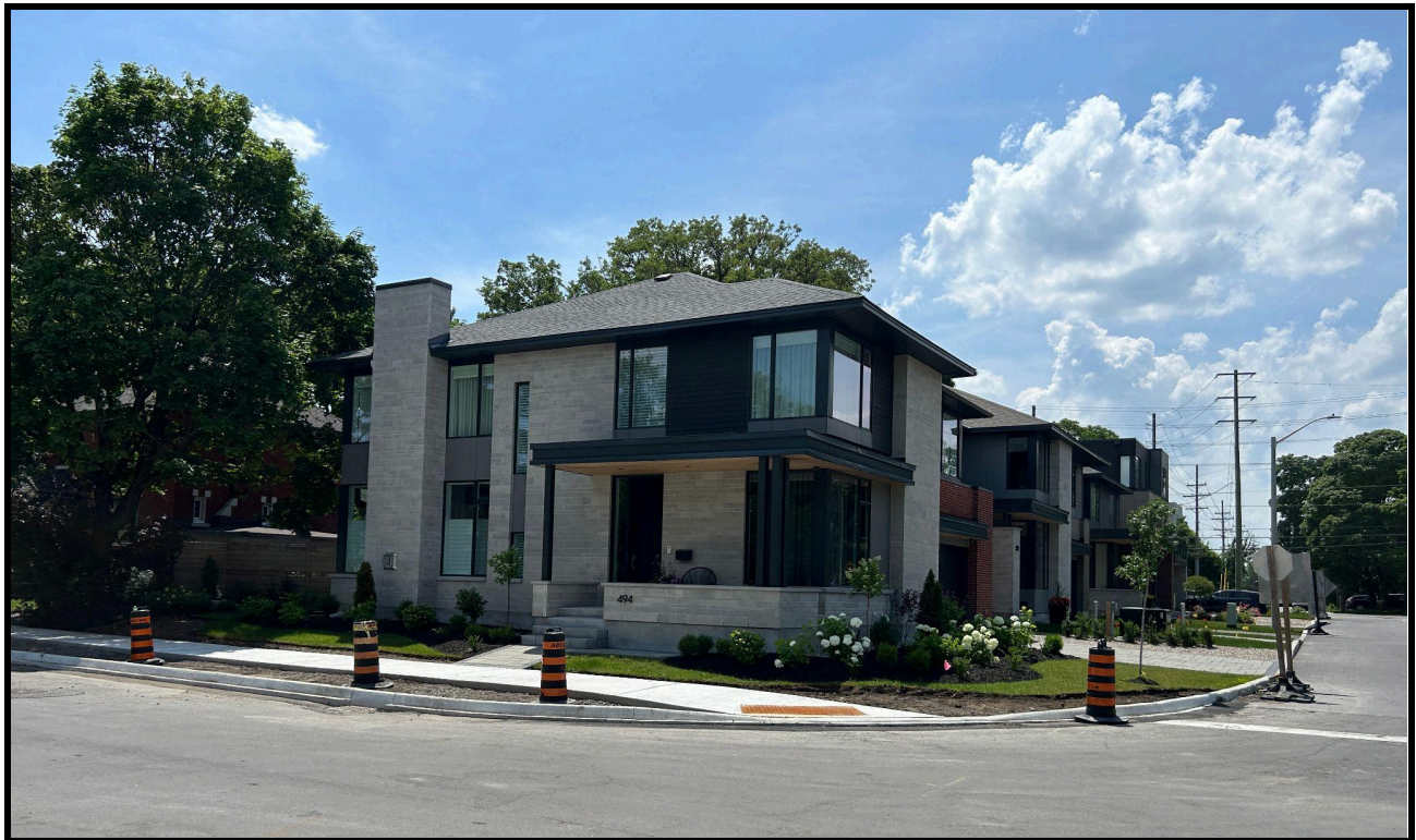
Newly constructed semi-detached dwellings at 494 Highcroft and 320 Kenwood.
