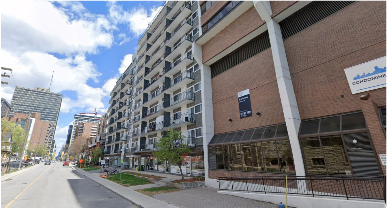
Figure 3: The south side of Queen Street, with 434 and 424 Queen Street in the foreground and the three single-detached buildings in the background.
