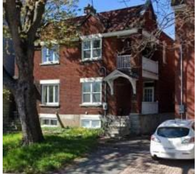
Figure 2: 454 & 456 Nelson Street: As seen from North Right of Way courtesy of Google Street View.
