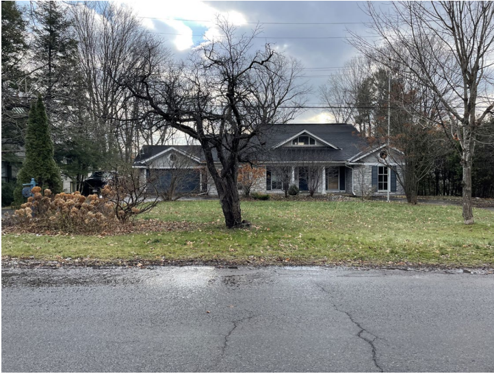
125 Lakeway Drive, Photograph taken from the Street
