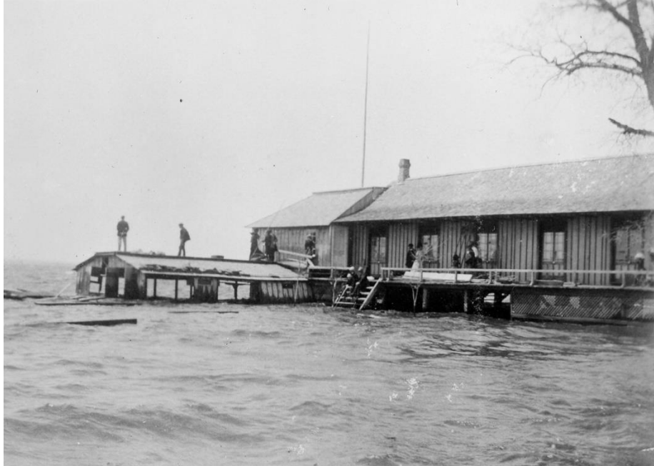
Flood waters at J. C. Jamieson's mill, Britannia, circa 1893, Source: City of Ottawa Archives, MG165-01-06, CA025473
