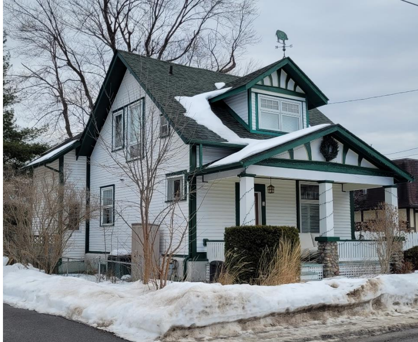
73 Britannia Road, west and north façade, Source: City of Ottawa, 2024
