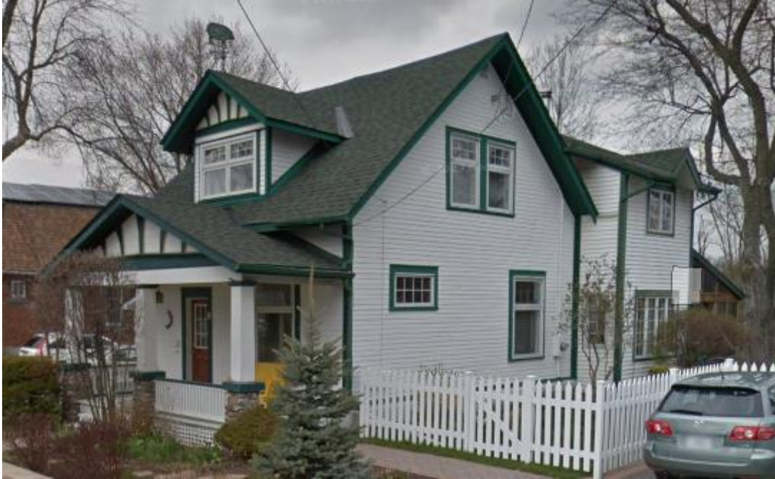
73 Britannia Road, west and south façade, Source: Google Maps, 2016
