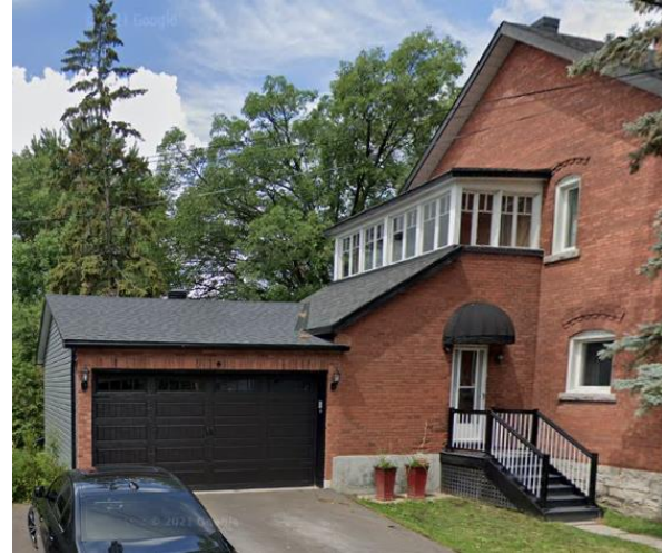
South façade, 2764 Rowatt Street, Source: Google Maps, 2021
