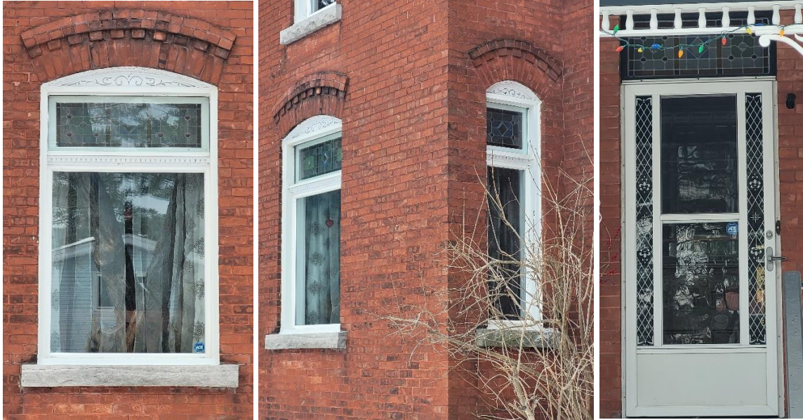
2764 Rowatt Street, flat transoms with stained glass windows on first floor windows and above main door, Source: City of Ottawa, 2024
