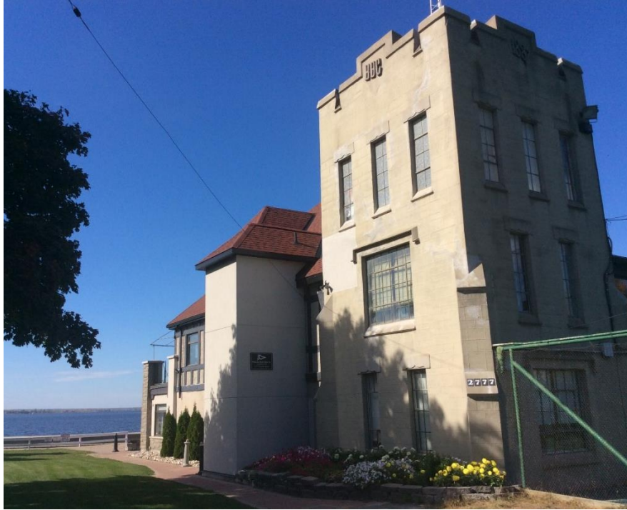
Southeast corner, 2777 Cassels Street, Source: City of Ottawa, 2016
