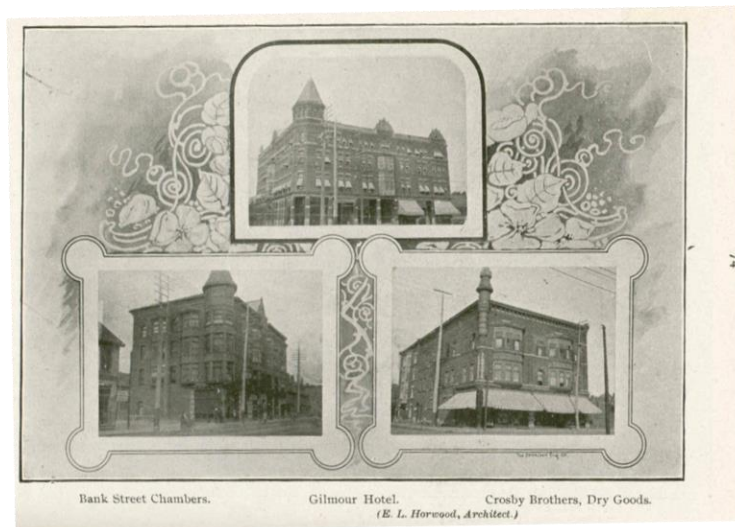
Bank Street Buildings, Source: Gard, The Hub and the Spokes , "The Old Art Gallery," 74.
