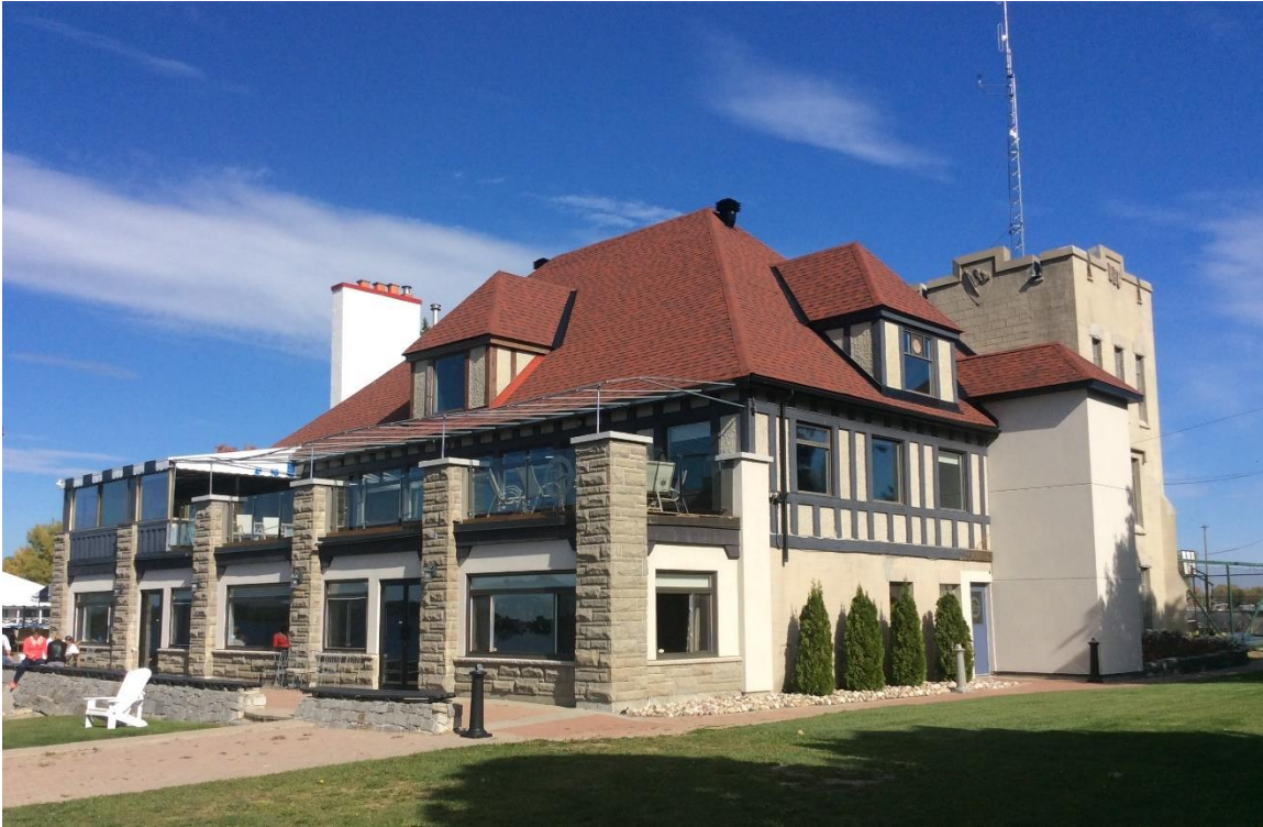
Southwest corner, 2777 Cassels Street, Source: City of Ottawa, 2016
