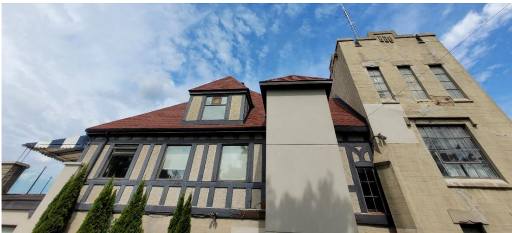
South façade, 2777 Cassels Street, Source: City of Ottawa, 2023
