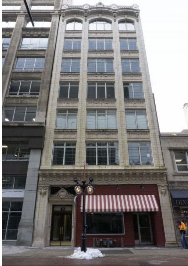
Saxe Building at 75 Sparks Street, Carleton University , 2020.
