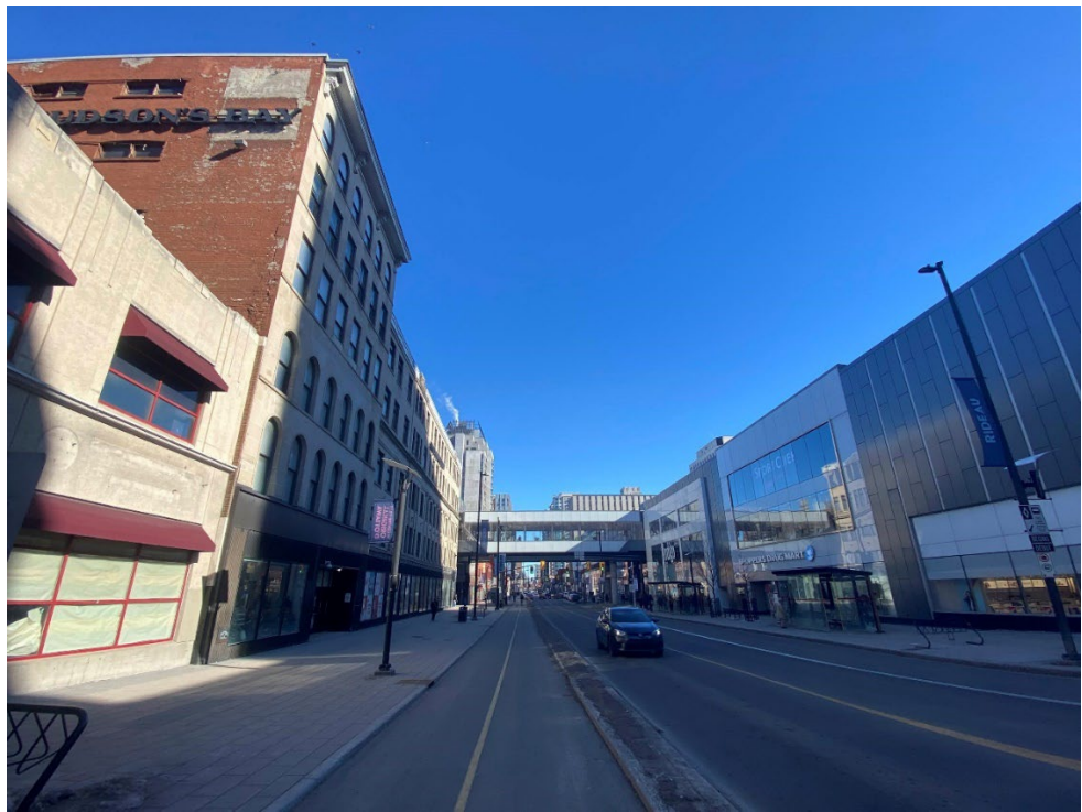
73 Rideau Street is integrated into the Rideau Centre. City of Ottawa, 2024.
