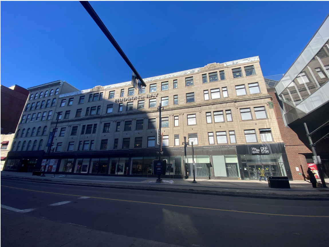
Front façade, City of Ottawa , 2024.
