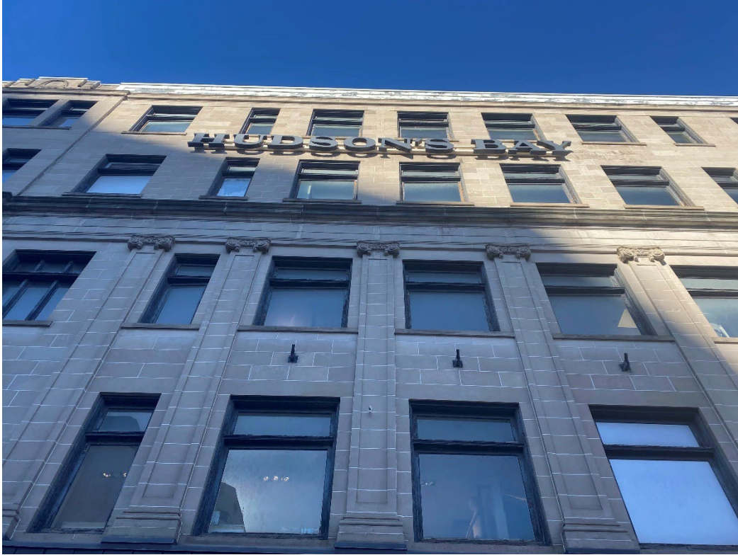
Shallow pilasters between windows on the second and third storeys. City of Ottawa, 2024.
