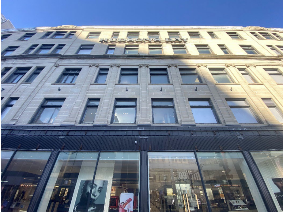
View of the repeating windows and string course. City of Ottawa, 2024.
