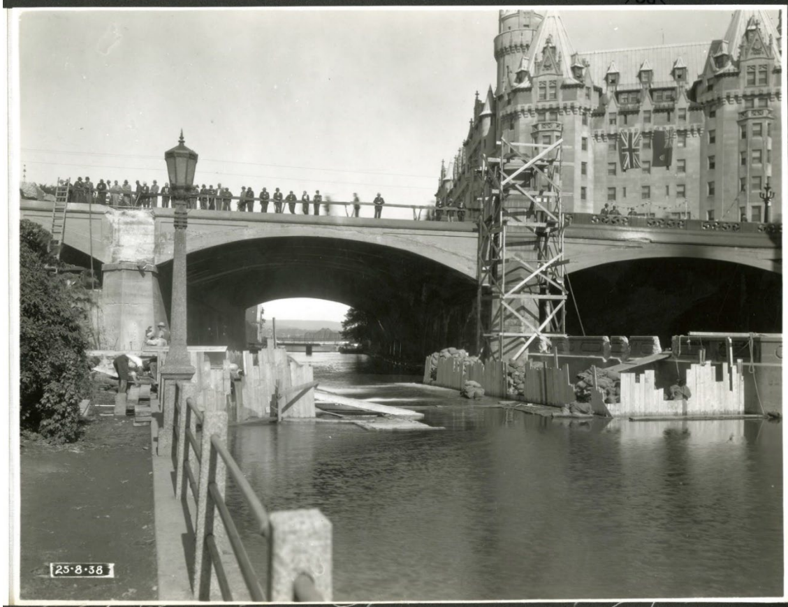
Plaza Bridge expansion, 1938.
