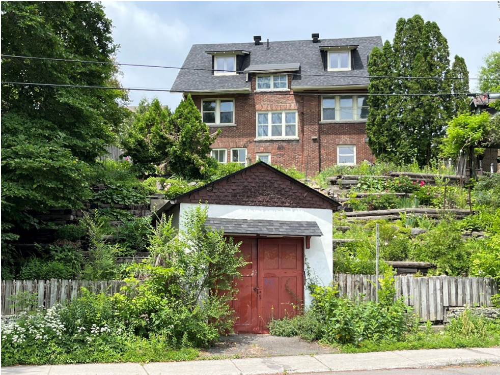
Rear (south) elevation facing Riverdale Avenue Source: City of Ottawa
