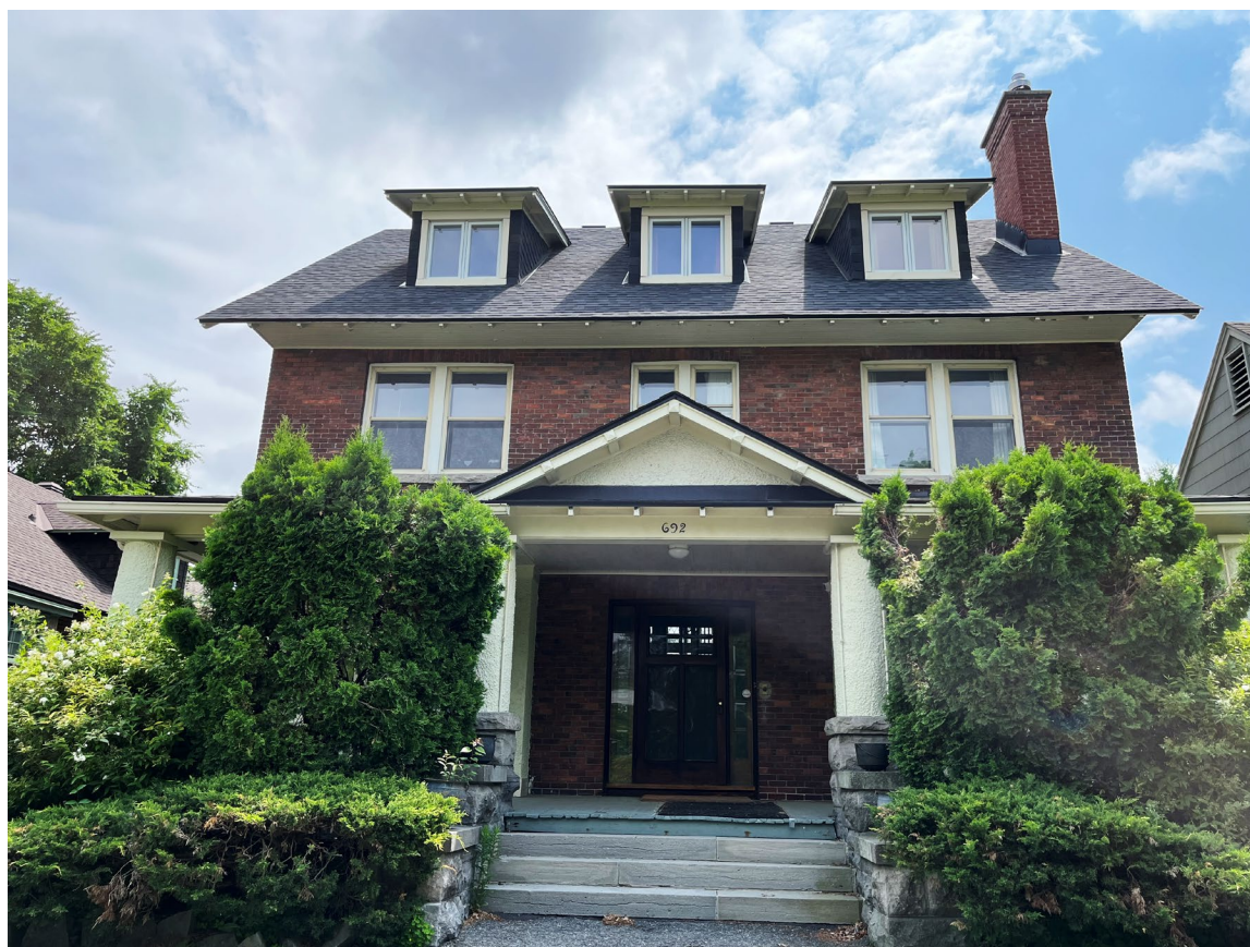
Front Façade Source: City of Ottawa, 2023
