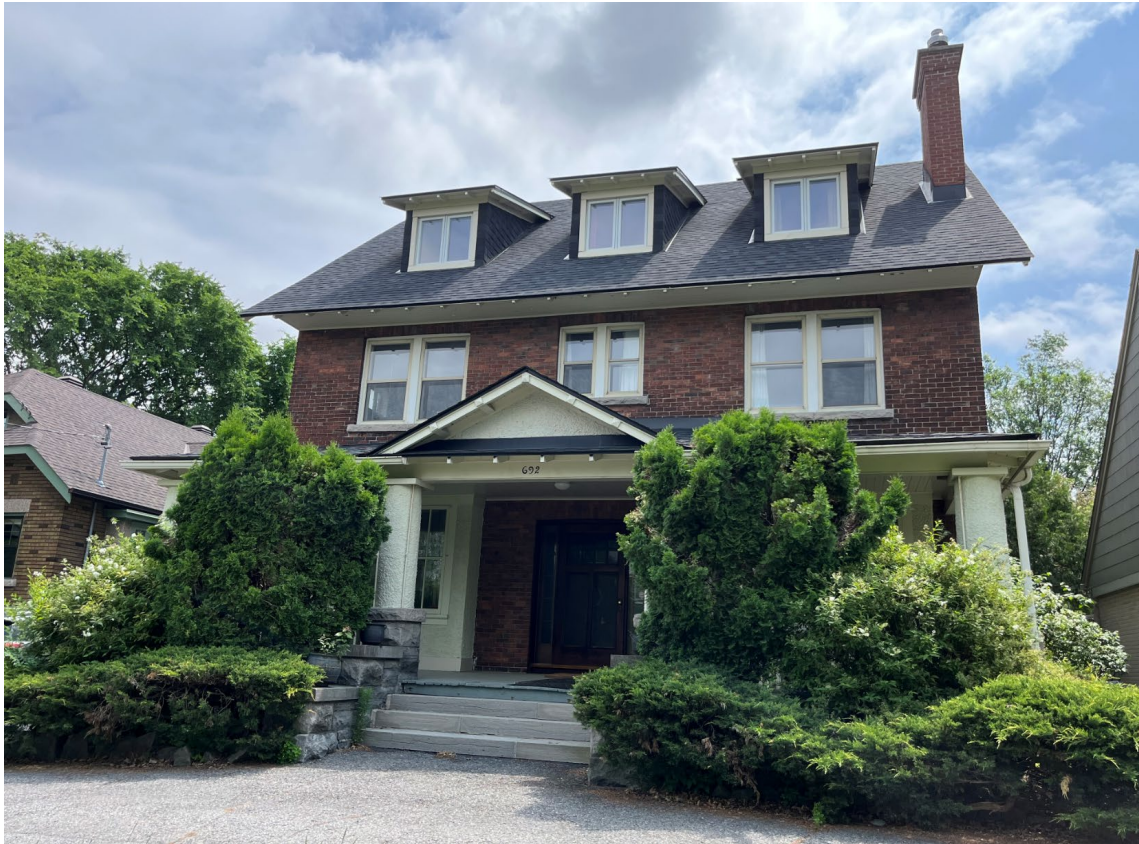
Front façade of 692 Echo Drive. Source: City of Ottawa
