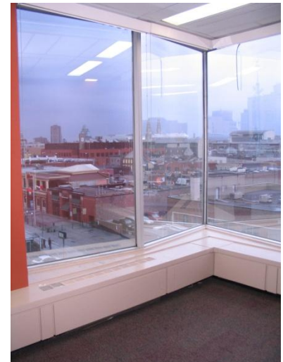
ANGLED WINDOW UNITS, NW CORNER OF BUILDING
