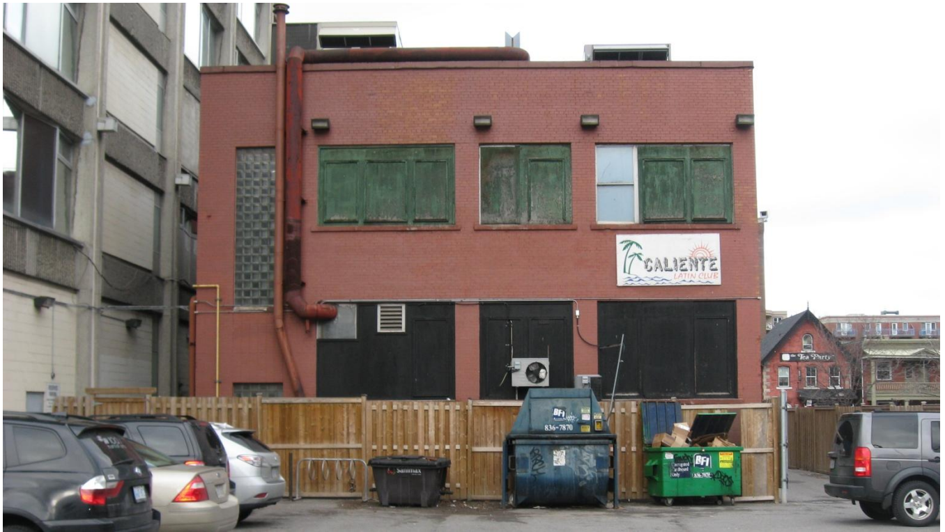
110 YORK, VIEW TO N (REAR WALL)
