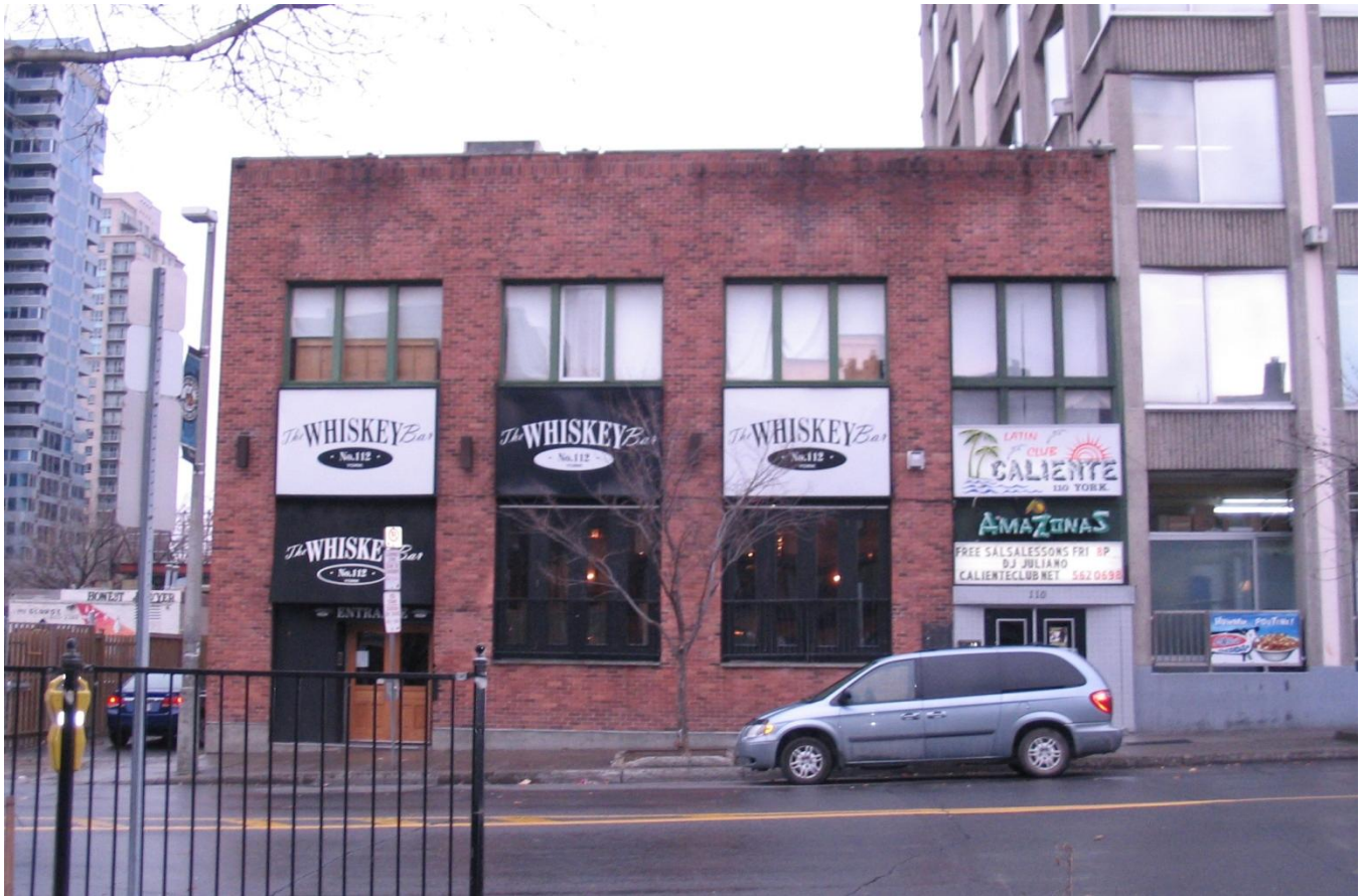
110 YORK, VIEW TO S (FACADE)
