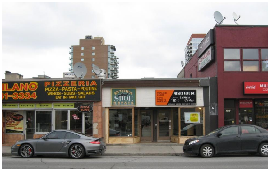
341-343 DALHOUSIE, VIEW TO E
