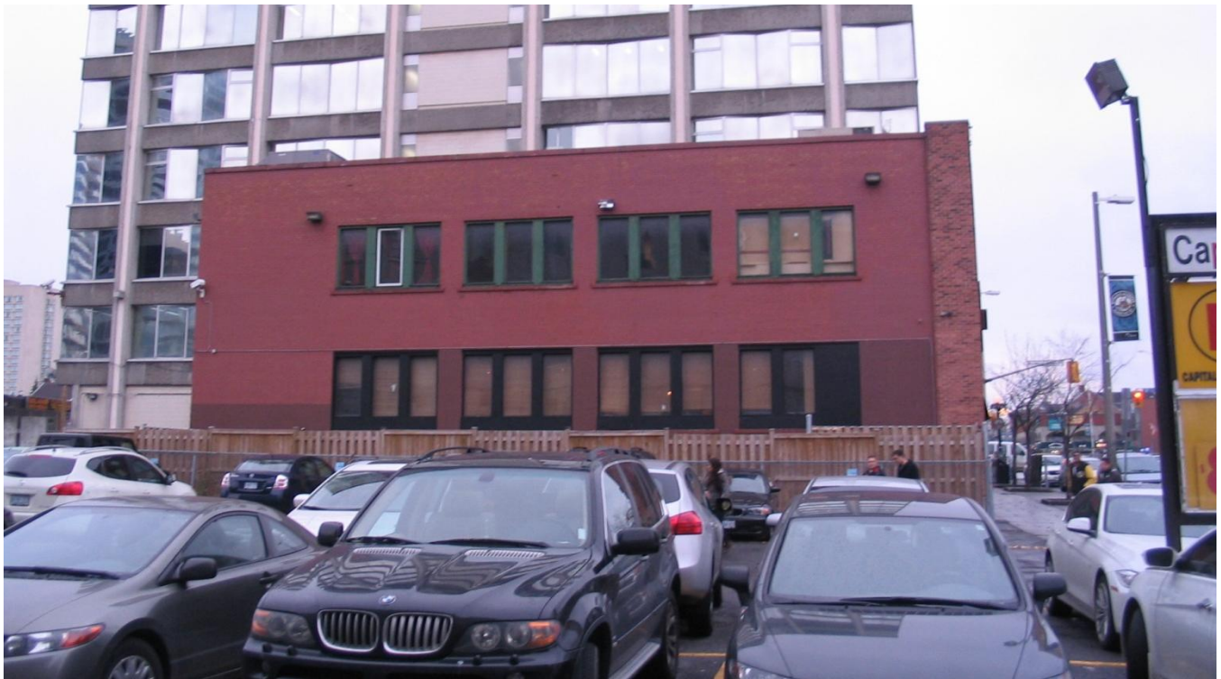
110 YORK, VIEW TO W (SIDE WALL)
