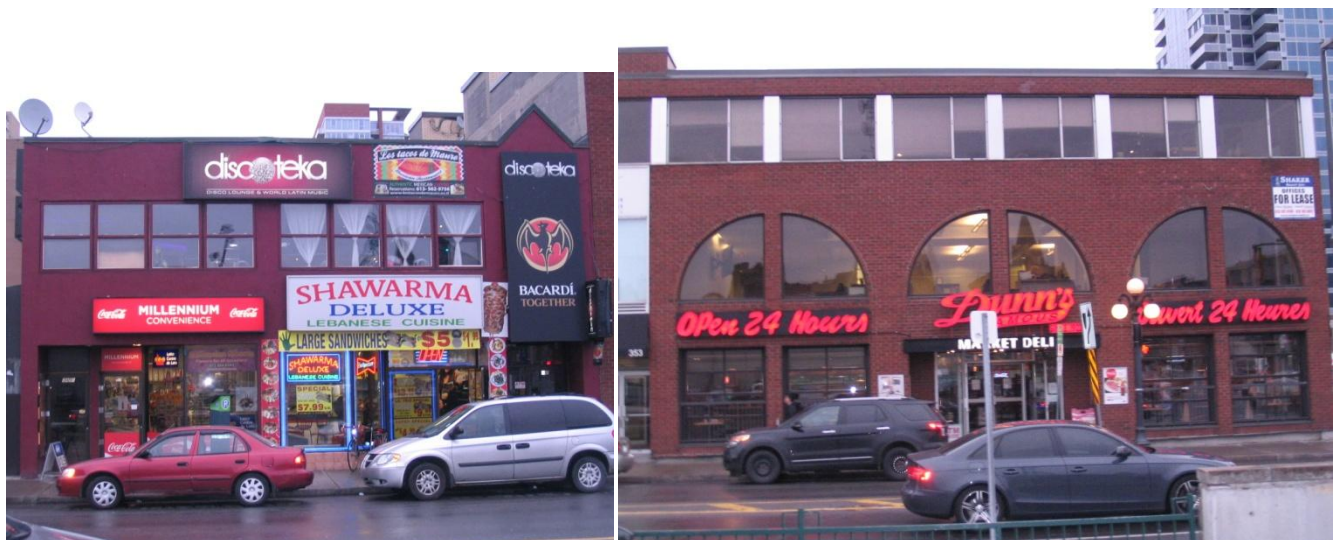
345-349 DALHOUSIE, VIEW TO E
