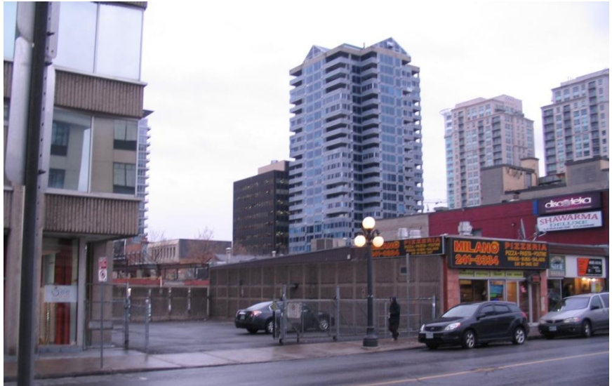
321 DALHOUSIE, VIEW TO SE OF SURFACE PARKING LOT ON DALHOUSIE
