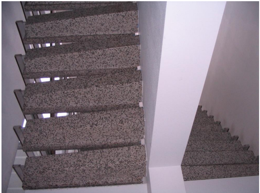
CANTILEVERED STAIRS ON S SIDE OF ENTRANCE LOBBY, FROM BELOW
