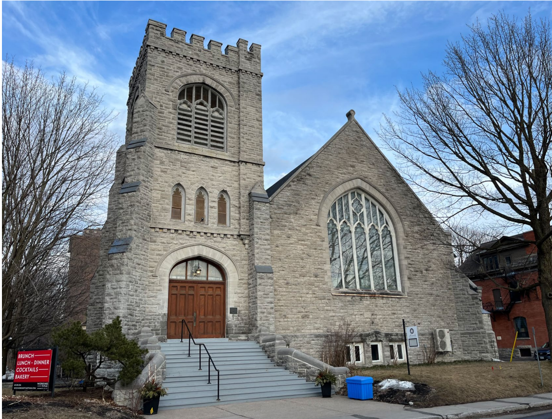
315 Chapel Street (former All Saints Anglican Church), front façade
