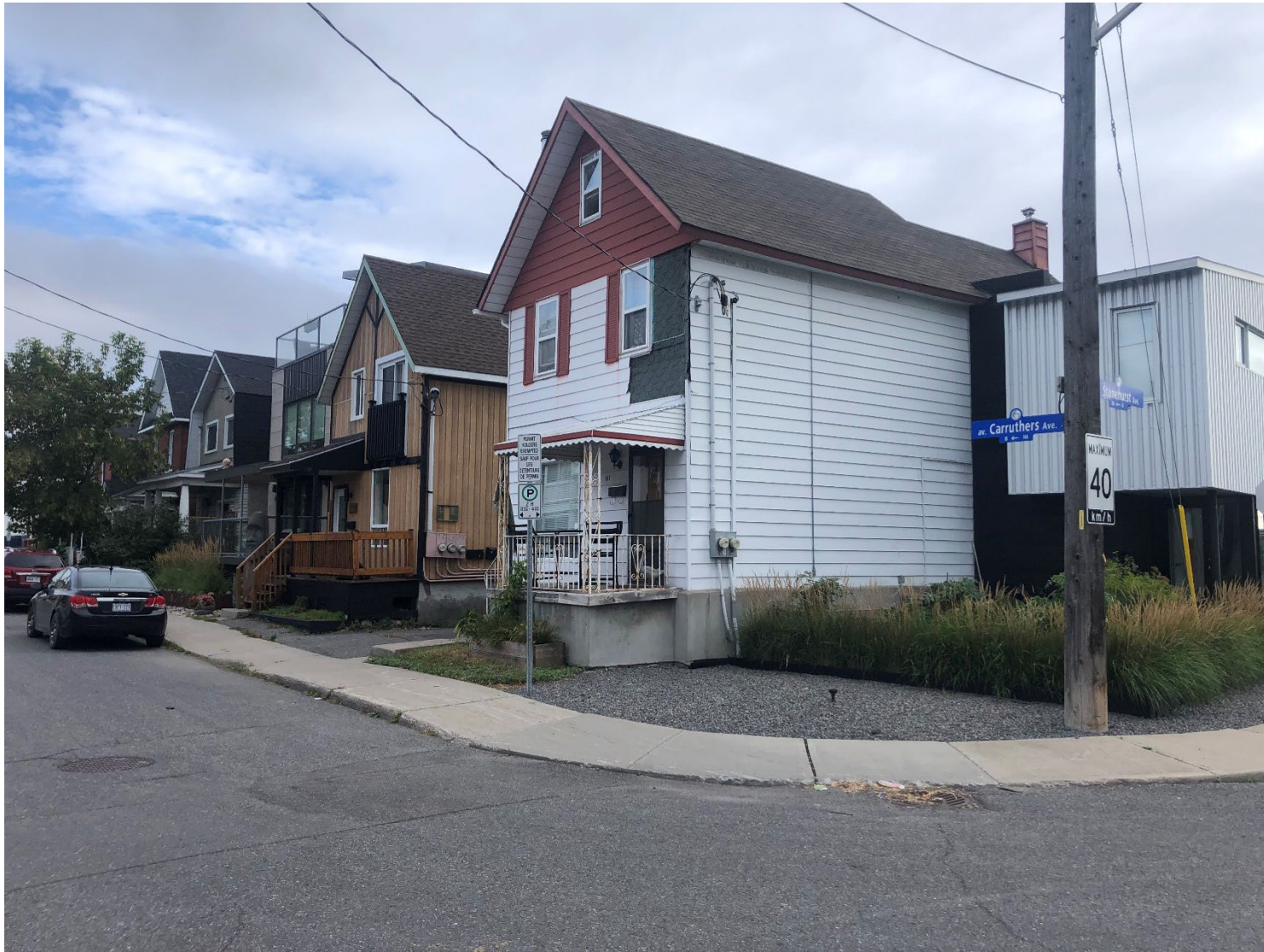
141 Carruthers Ave – Carruthers Avenue & Stonehurst Avenue existing conditions.
