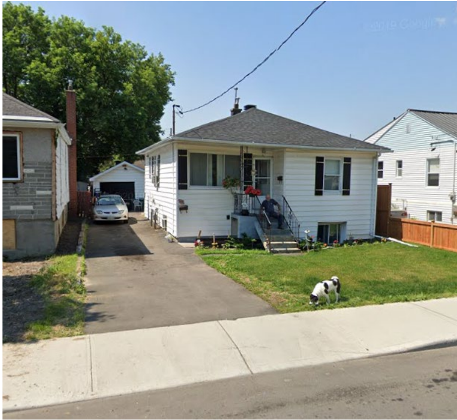
Figure 2 – Street view of 96 Joliet Avenue
