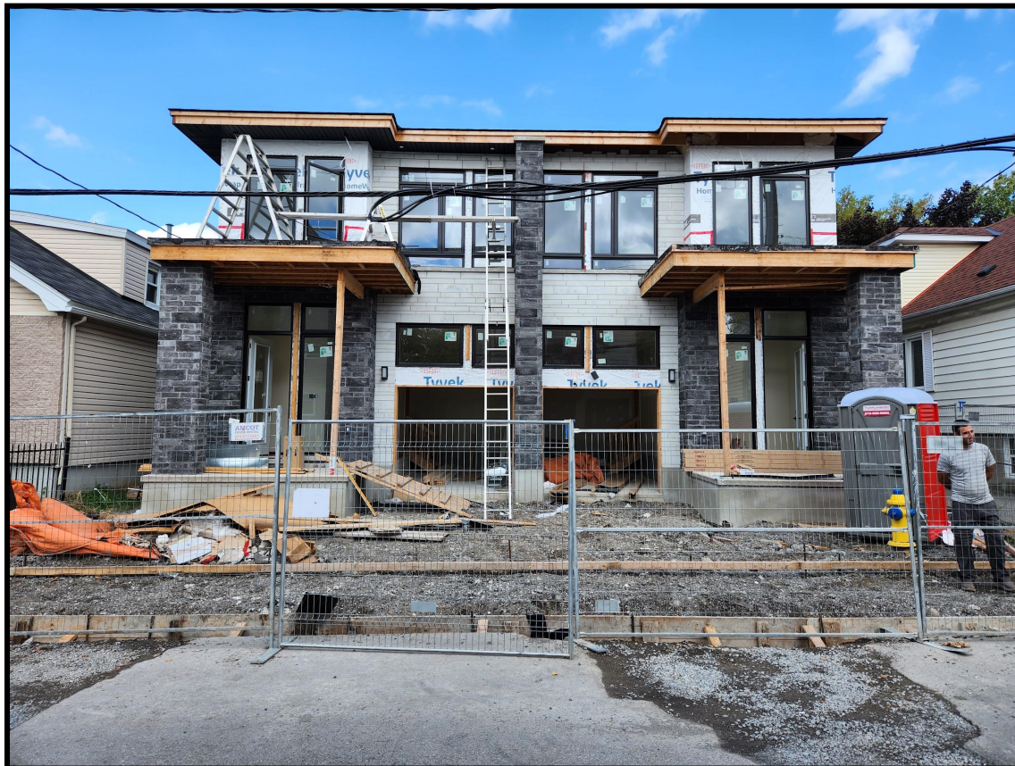
September 2023 imagery showing the semis under construction
