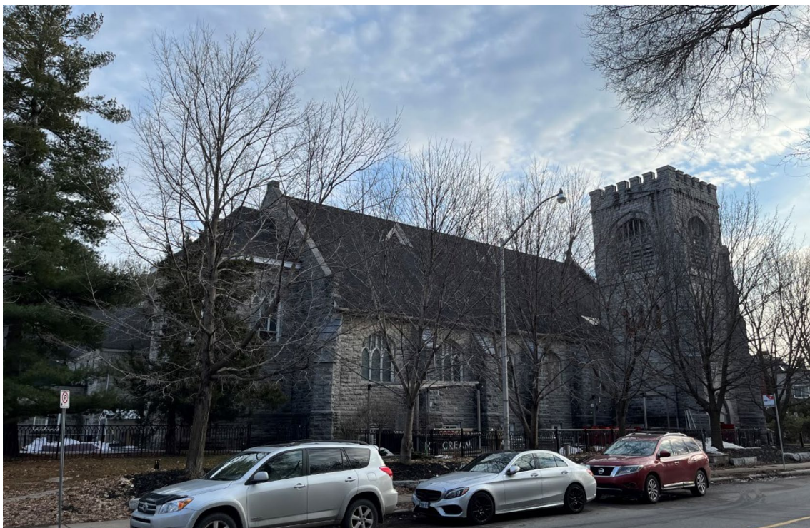
315 Chapel Street (former All Saints Anglican Church), side elevation along Laurier Avenue East
