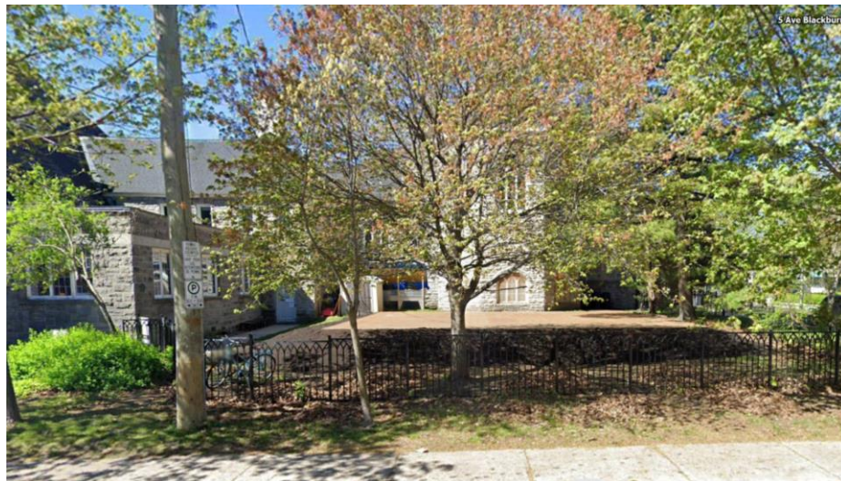
Figure 6: May 2021 Street view looking west to the apse of the church. Bate Memorial Hall is to the left. Note the landscape characteristics with a treed verge. Source: Google Earth
