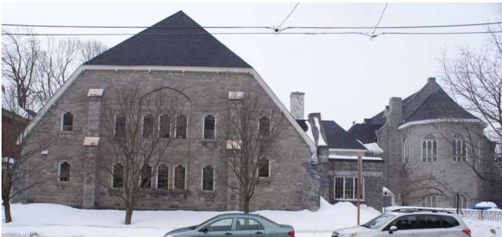
Figure 10: View of the Blackburn Avenue frontage with the 1934 Bate Memorial Hall (left) and the apse of the former All Saints Anglican Church (right). Source: Commonwealth 2023
