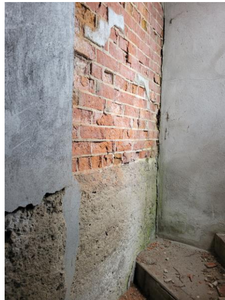
Brick Deterioration
