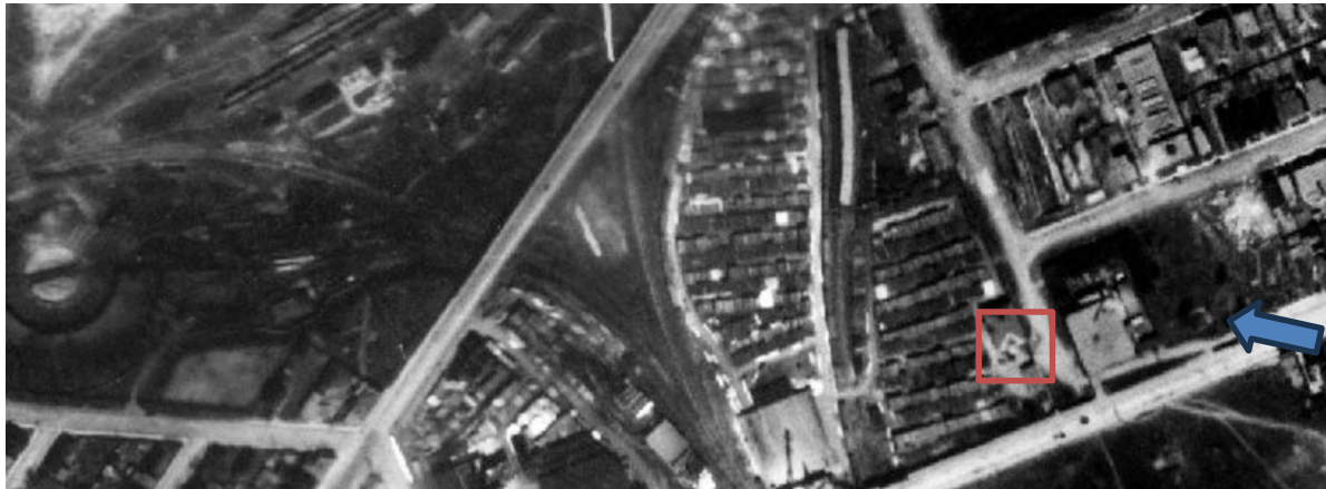
Figure 10: 1928 aerial view of the W. C. Edwards Co. lumberyard. The building fronted on to Somerset Street, with
