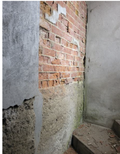
Brick Deterioration
