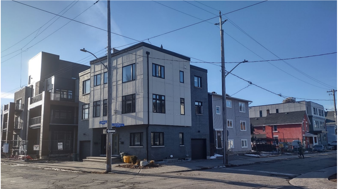
Figure 3. Looking northwest at the corner of Armstrong Street and Carruthers Avenue. The building under construction at 177 Armstrong Street can be seen on the left of the image and 266 Carruthers Avenue can be seen on the right side of the image (red building).
