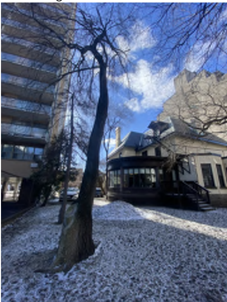
c leaning SW toward addition area
