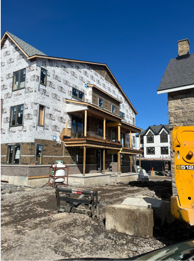
Figure 8: Photograph of the balconies as constructed
