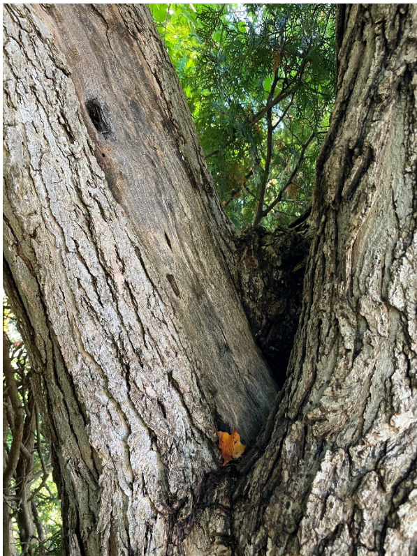
Figure 2: Decay in junction of tree 1
