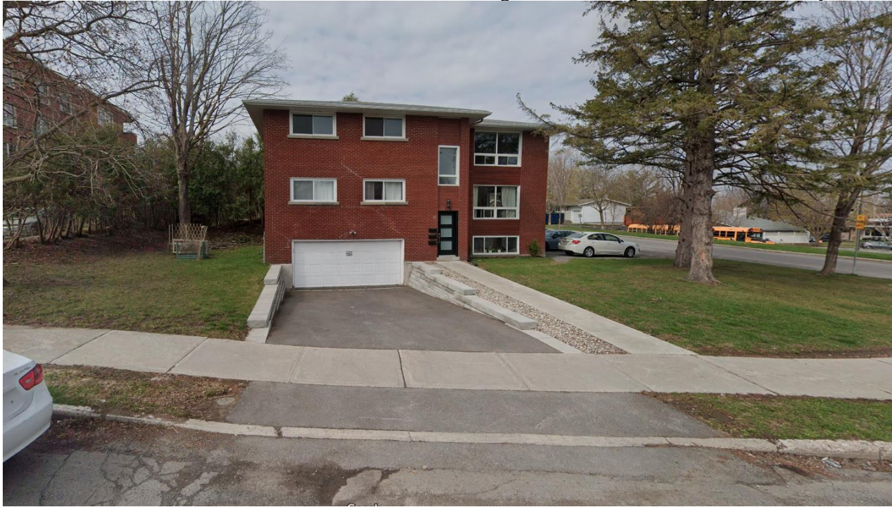
Figure 3: Existing Building on the Subject Site
