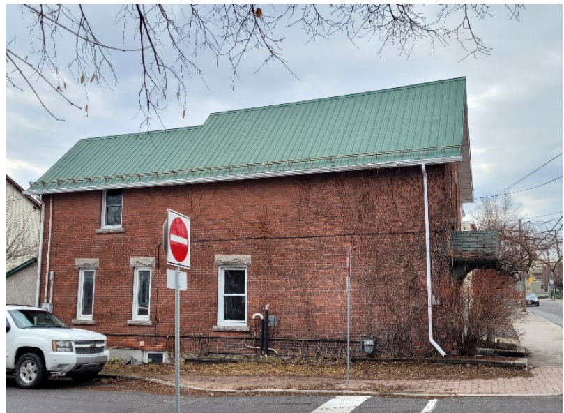
North facade, 241 Marier Avenue, Source: City of Ottawa, 2024
