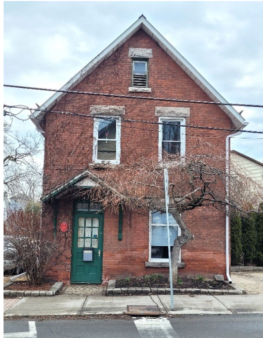
Front façade, 241 Marier, Source: City of Ottawa, 2024
