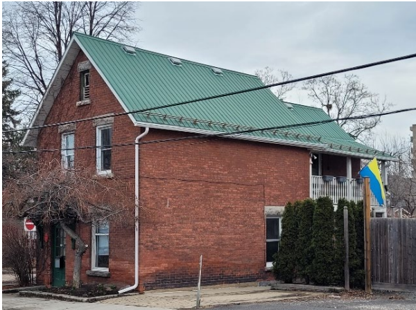
West and south façades, 241 Marier Avenue, Source: City of Ottawa, 2024
