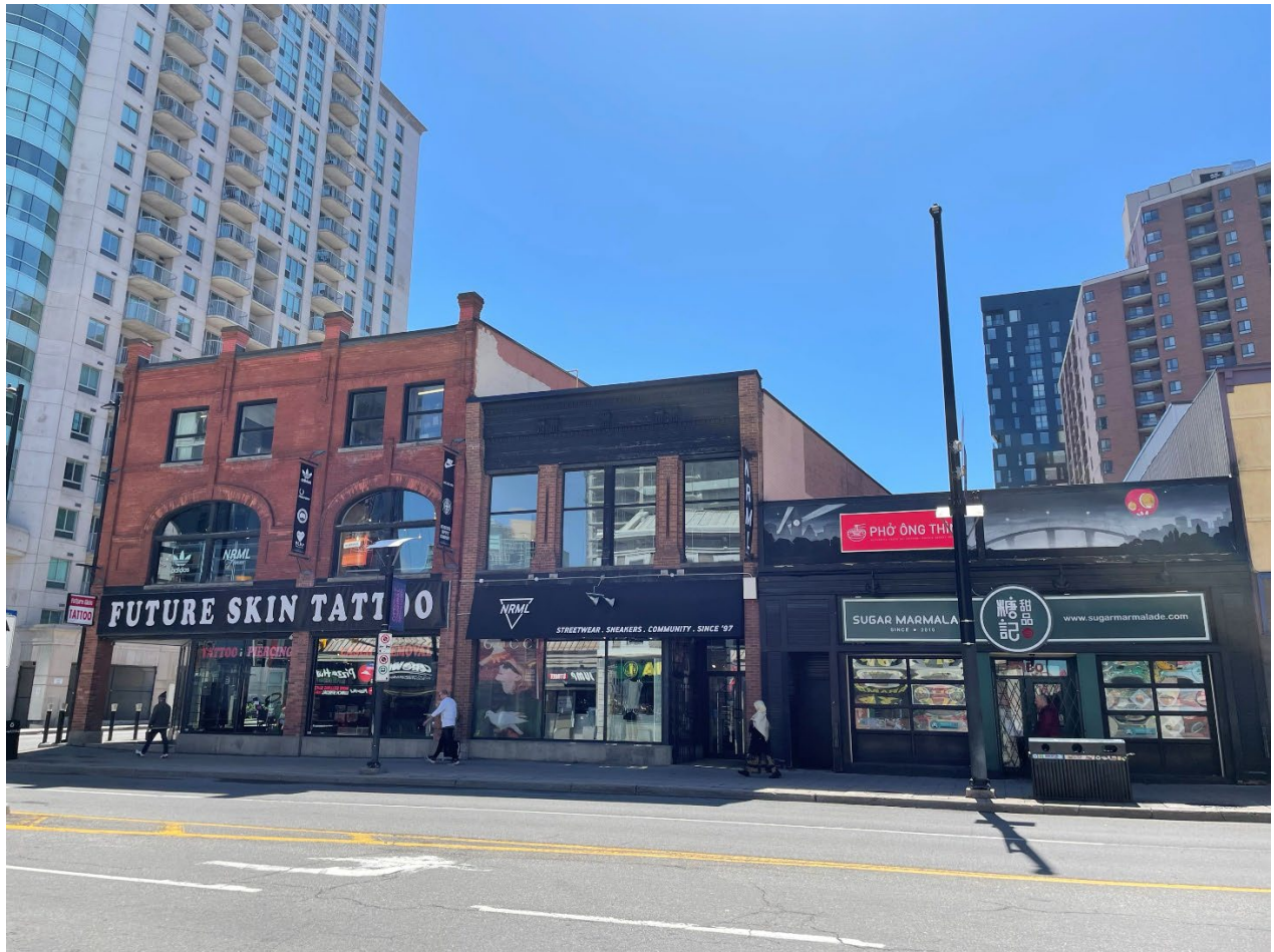
198 Rideau Street show the Rideau Street façade. City of Ottawa, 2024.
