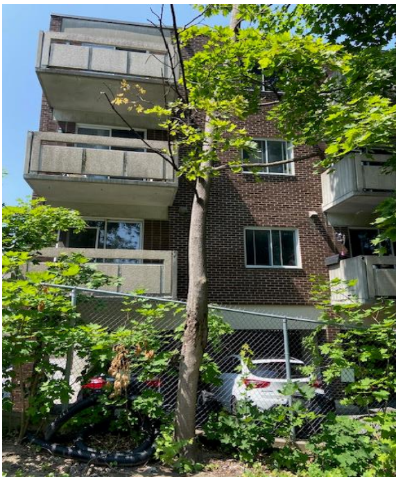
Tree #5, 814 High st, Norway Maple with rotten area on main trunk, to be removed.
