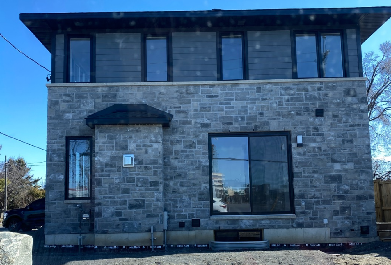
Image 2. Semi-detached under construction, looking south from corner of Louis Lane
