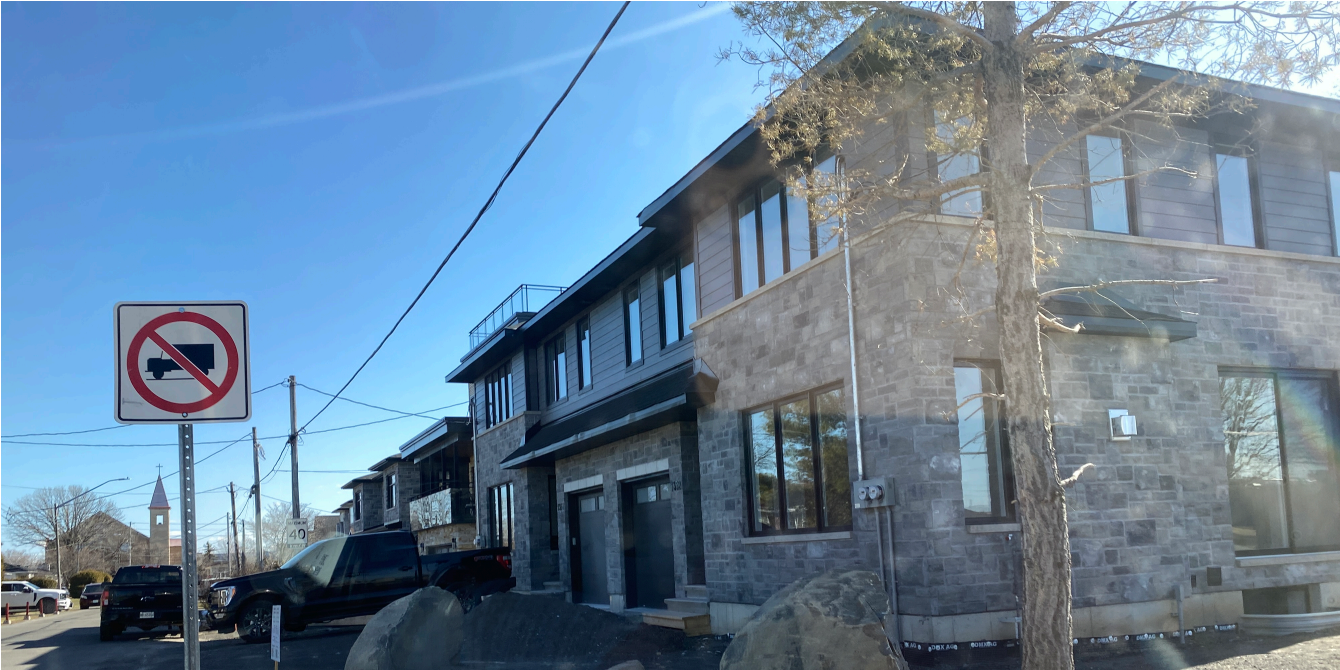
Image 1. Semi-detached under construction, looking from corner of Louis and Parisien
