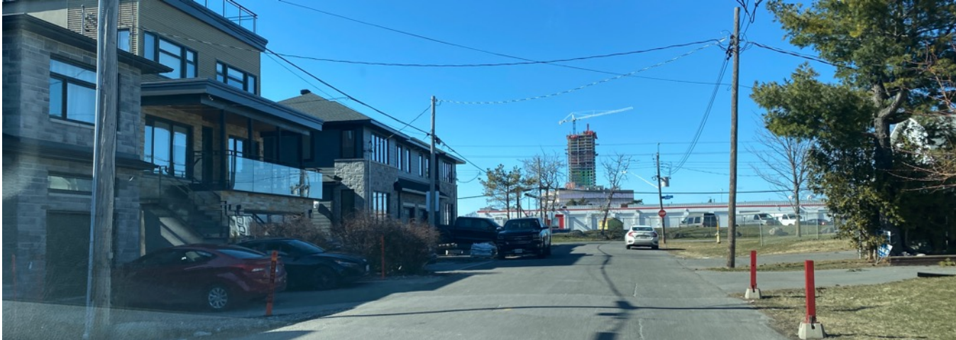
Image 3. Semi-detached under construction and surrounding dwellings, looking north from Louis Lane
