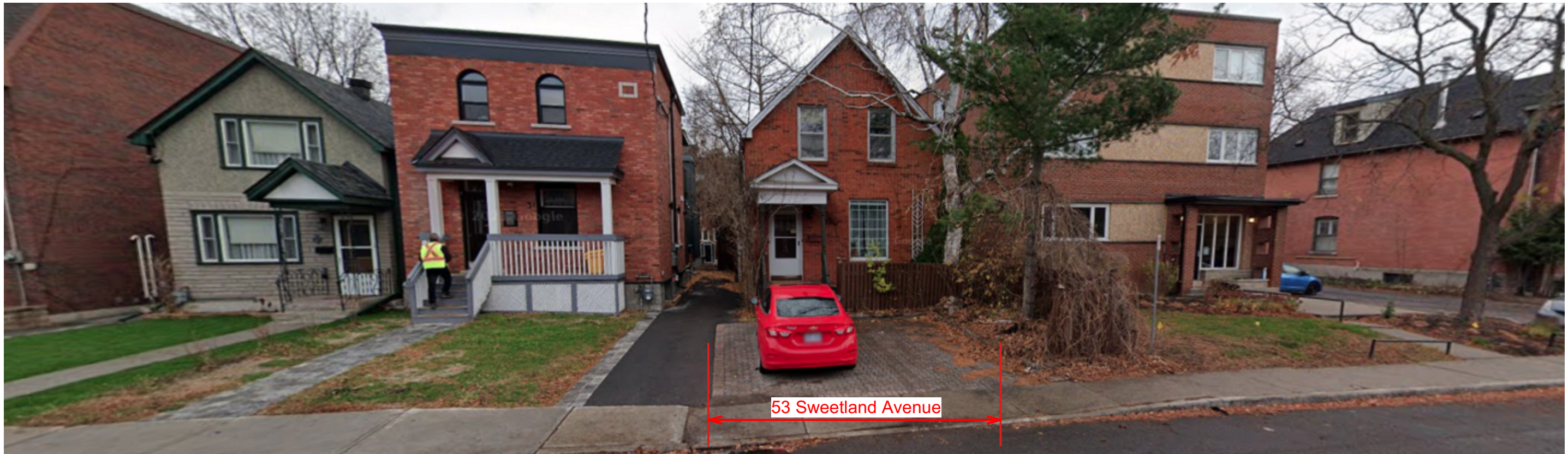
A) Exterior photo of subject property 53 Sweetland Avenue between neighbouring buildings 51 Sweetland Avenue and 55 Sweetland Avenue.
