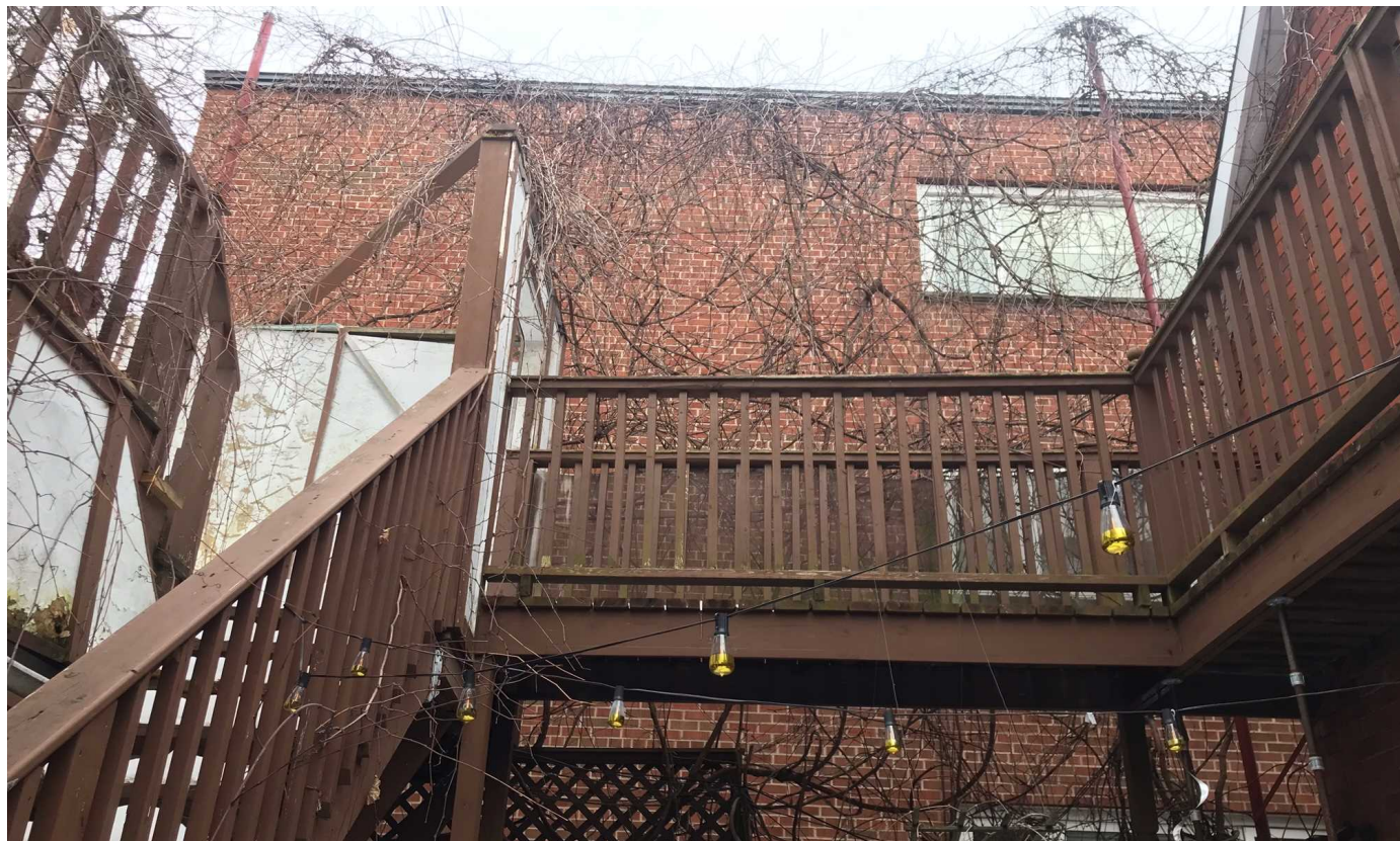
S) View of the elevated walkway and 55 Sweetland Avenue behind from the courtyard.
