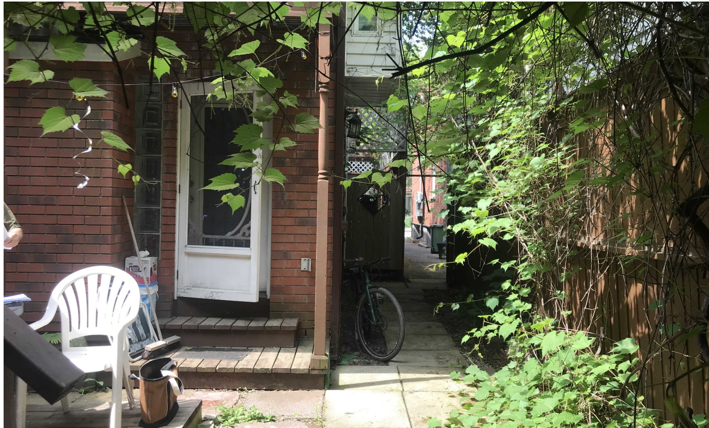
D) View of the rear unit's exterior access and entrance looking towards Sweetland Avenue.
