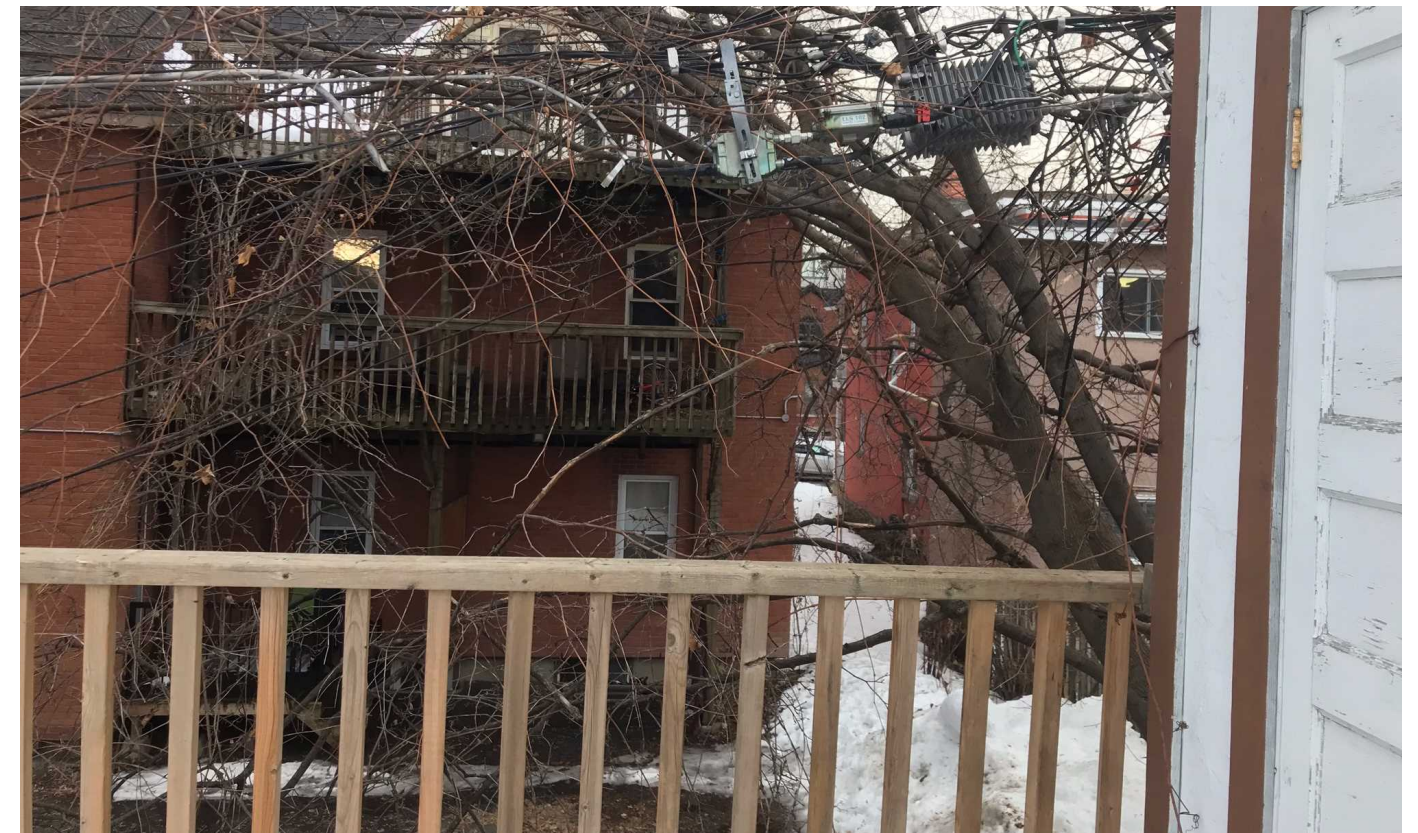
P) View of the neighbouring recessed balconies (50 Russell Avenue) from the roof deck.
