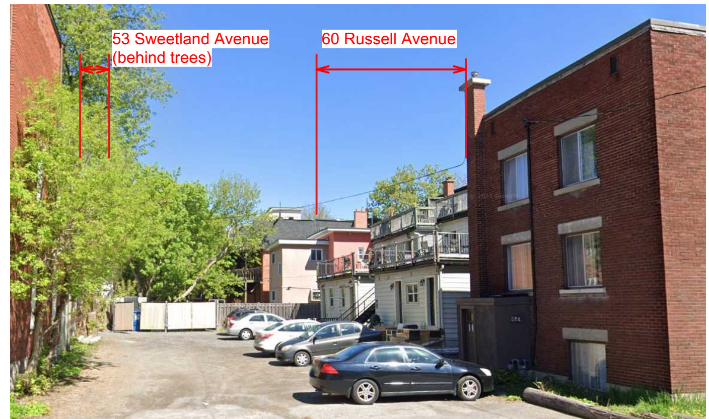
C) View of the parking lot and rear balconies at 60 Russell Avenue from Osgood Street.
