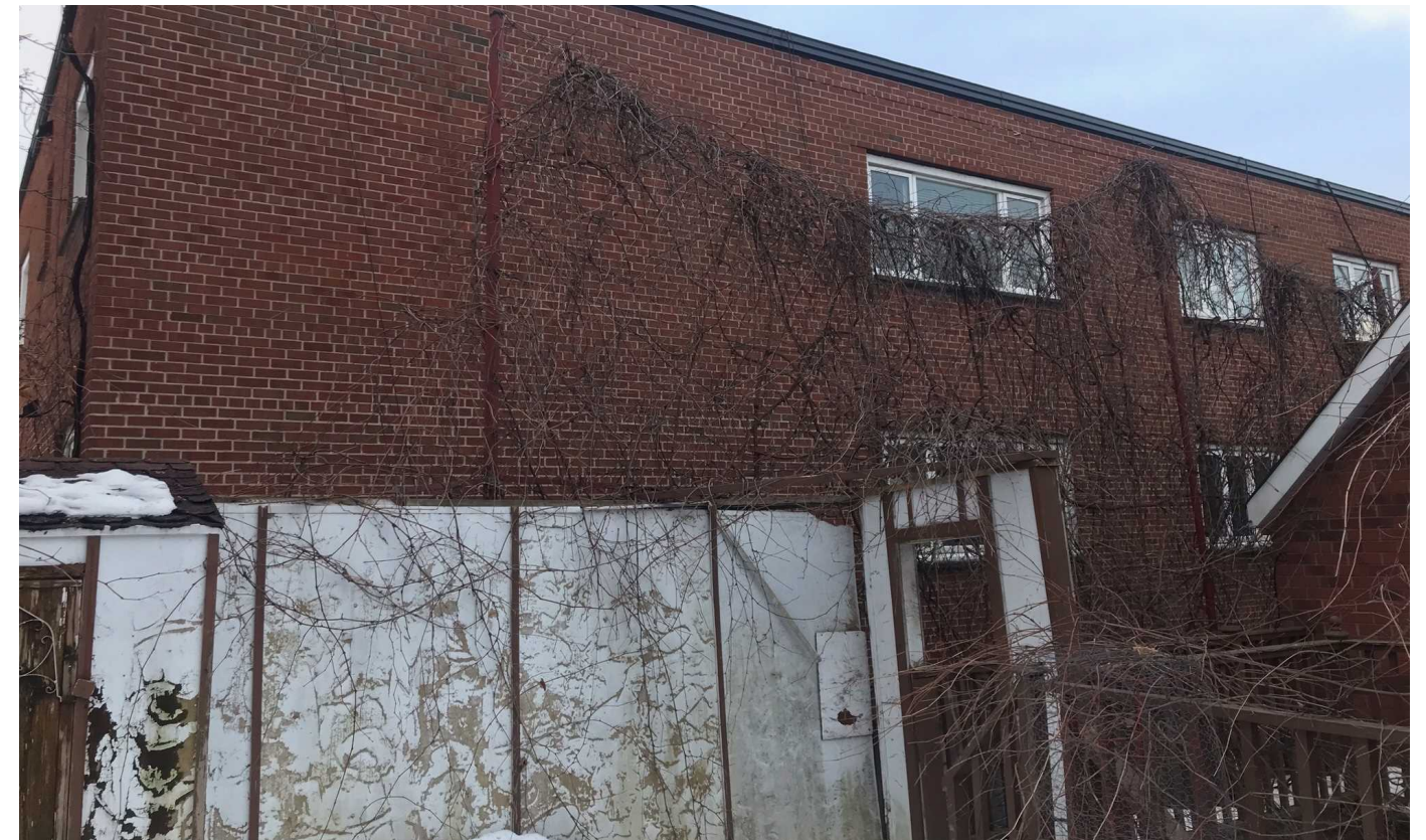
R) View of the 55 Sweetland Avenue from the roof top deck.
