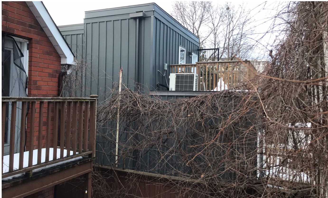
Q) View of the neighbouring roof top patio & condenser unit at 51 Sweetland Avenue from the elevated walkway of the subject property.
