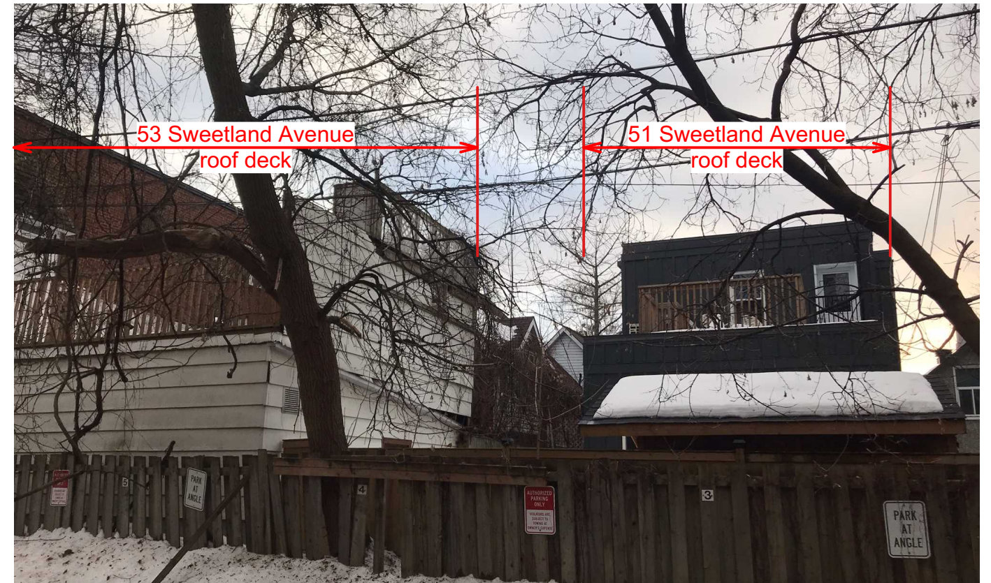
N) View of the roof top decks at 53 Sweetland Avenue and 51 Sweetland Avenue from 50 Russell Avenue.
