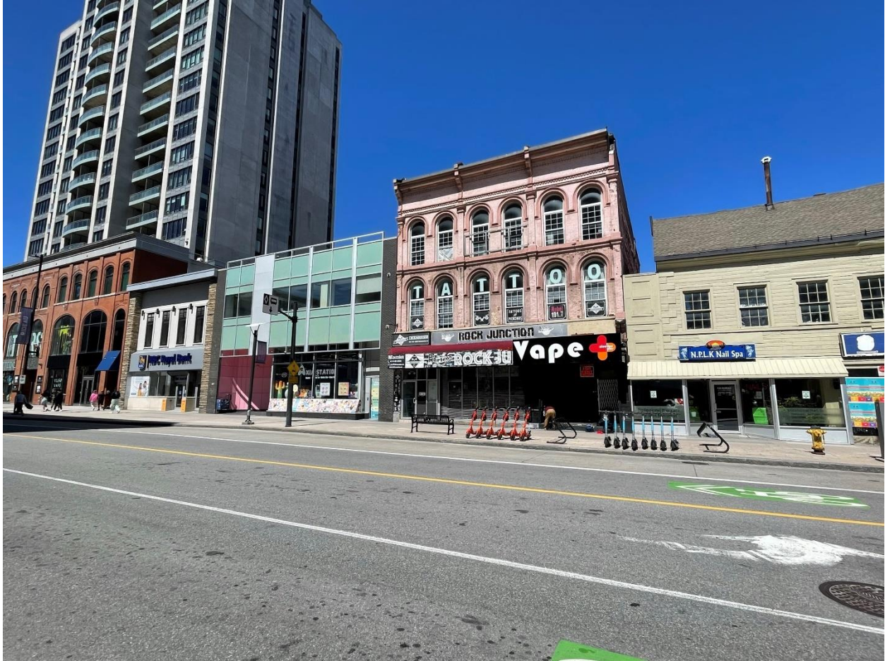
149 and part of 155 Rideau Street, on the north side of Rideau Street across from 152 and 156 Rideau Street. City of Ottawa , accessed 2024.
