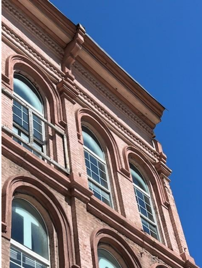
Large cornice on 149 Rideau Street, City of Ottawa , 2024.
