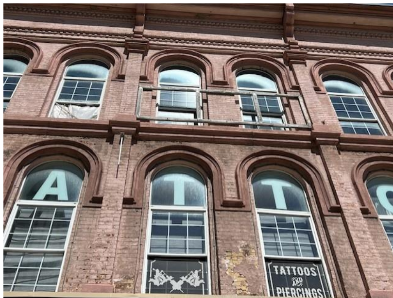
Continuous hooded stone moulding over the windows at 149 Rideau Street, City of Ottawa , 2024.
