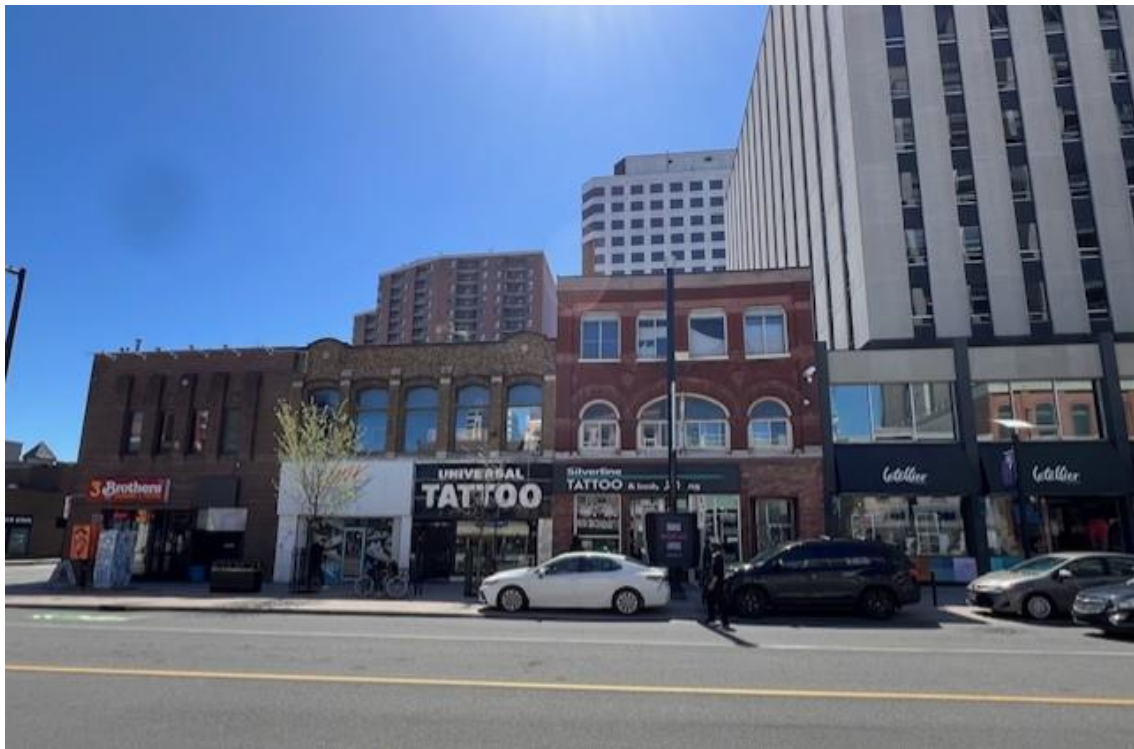
152 and 156 Rideau Street, on the south side of Rideau Street. City of Ottawa , 2024.
