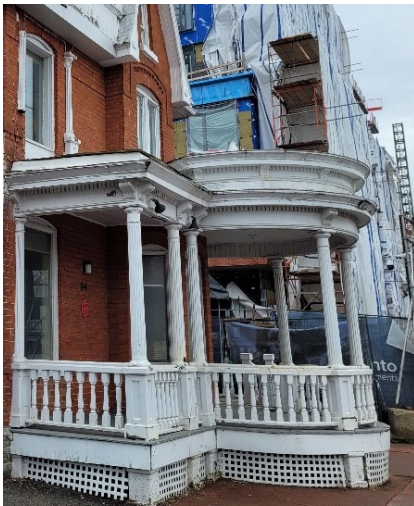
Front façade porch, 94 Beechwood Avenue, Source: City of Ottawa, 2024
