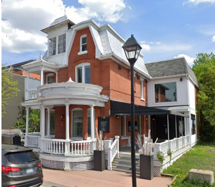
North and west facades, 94 Beechwood Avenue, Source: GoogleMaps, 2023
