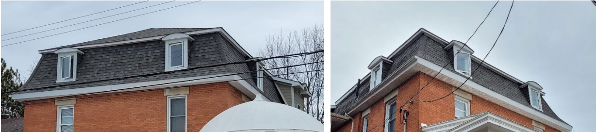
275 St. Laurent Boulevard, mansard roof on south, west, and north façades, Source: City of Ottawa, 2024
