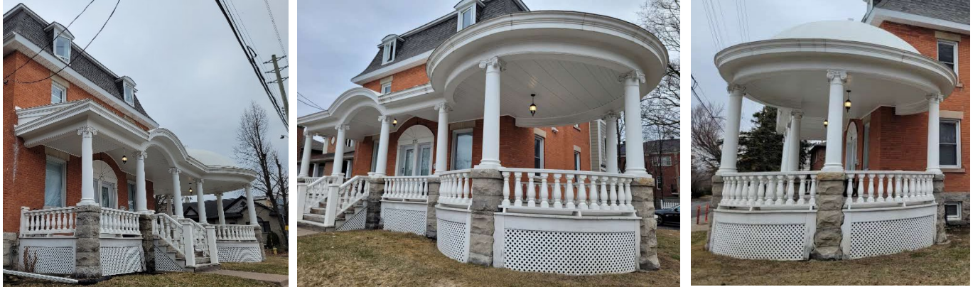
275 St. Laurent Boulevard, porch across front façade, Source: City of Ottawa, 2024
