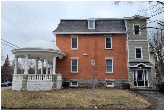
275 St. Laurent Boulevard, south façade, Source: City of Ottawa, 2024
