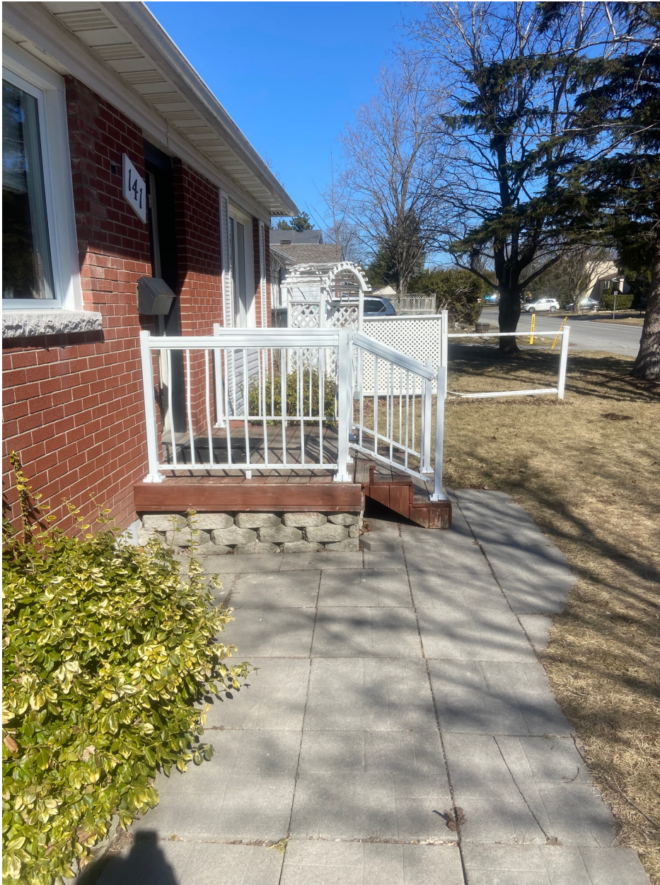
Image 1. Existing front steps.
