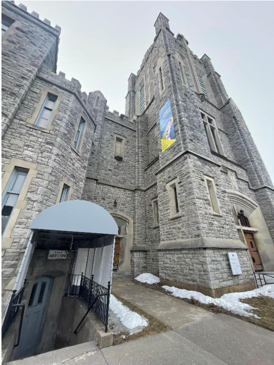
Bell tower and three-sided bay at 90 Primrose Avenue and 96 Empress Avenue
