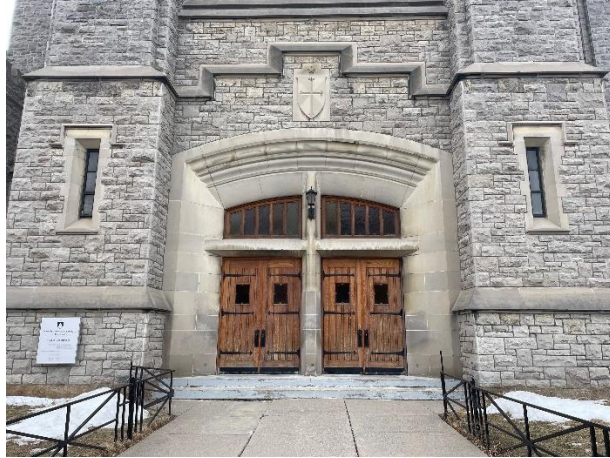
Main entranceway of 90 Primrose Avenue
