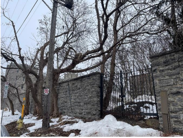
Stone wall with wrought iron gate from Upper Lorne Avenue
