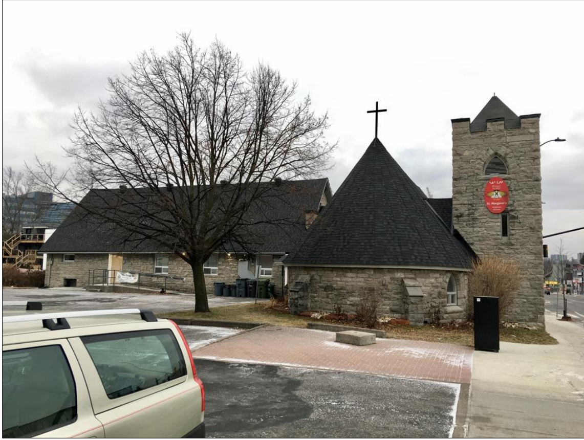
206 Montréal Road. East façades and parking area.
