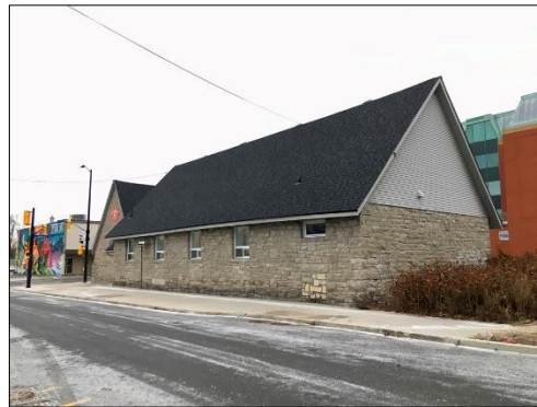
206 Montréal Road. West and south façades.
