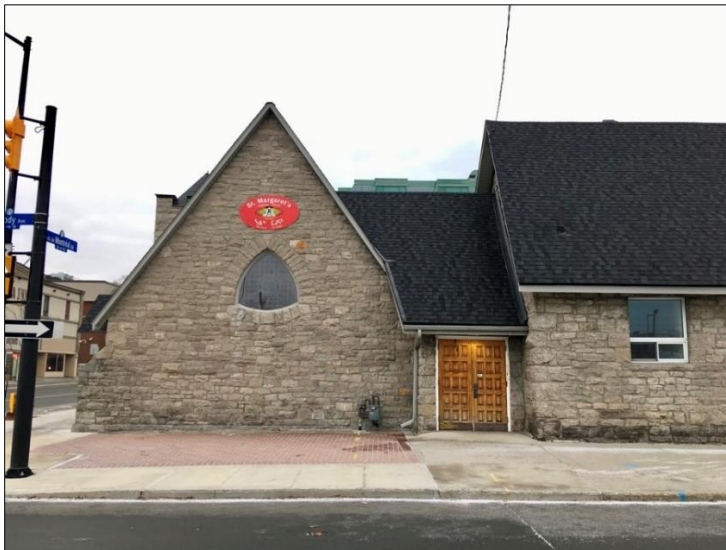
206 Montréal Road. Detail of west facade.
