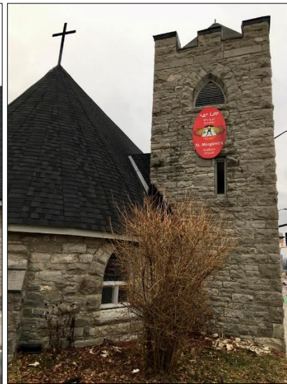
Detail of tower and curved apse.
