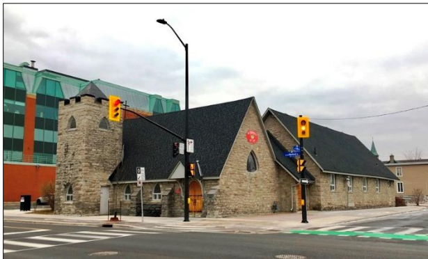
206 Montréal Road. North and west façades.
