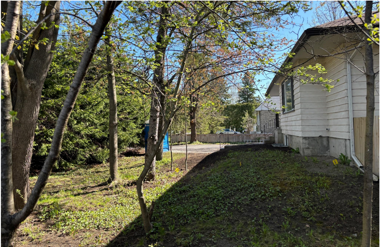
Figure 12, Retained dwelling at the corner of Moodie Drive and Anwatin Street
