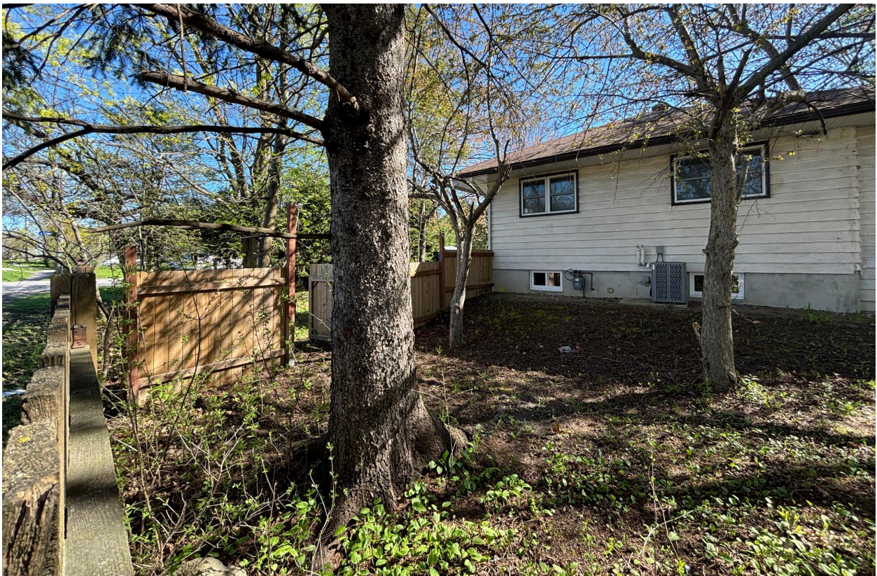
Figure 10, Retained dwelling at the corner of Moodie Drive and Anwatin Street
