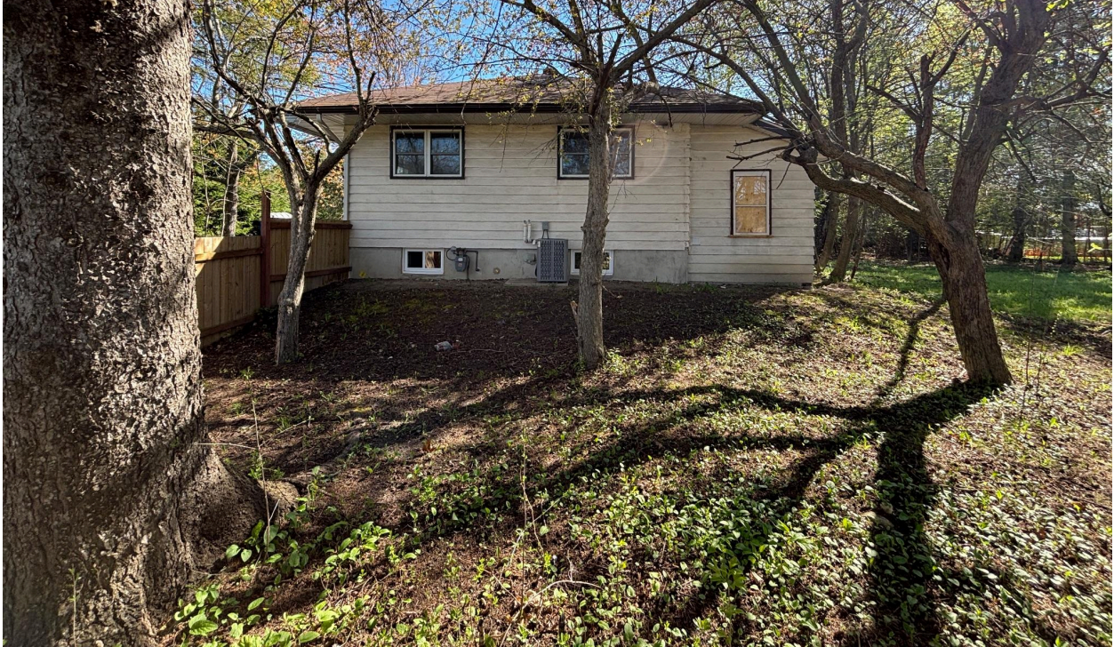
Figure 11, Retained dwelling at the corner of Moodie Drive and Anwatin Street
