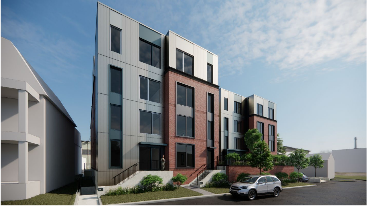
10 EMPRESS AVENUE VIEW FROM PERKINS STREET | 2014 | SCALE: NTS Project Studio Incorporated | mail@projectstudio.ca | projectstudio.ca
