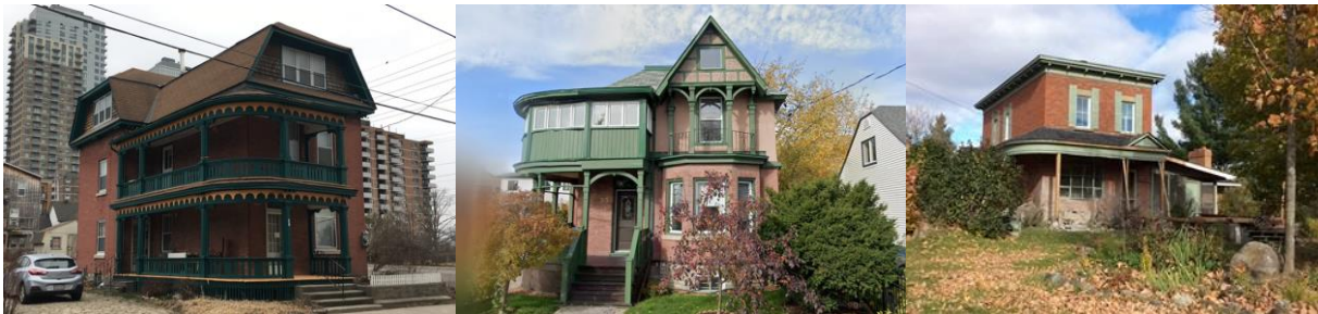
Left: Subject property, 50 Carruthers Avenue in Mechanicsville. Centre: 39 Queen Mary Street, Overbrook, near the Rideau River. Image: Oct 2020 © Google. Right: 5929 Buckland Road in Vars. Although its veranda is only one level, it expresses a similar curve. Image: 2018, City of Ottawa.
