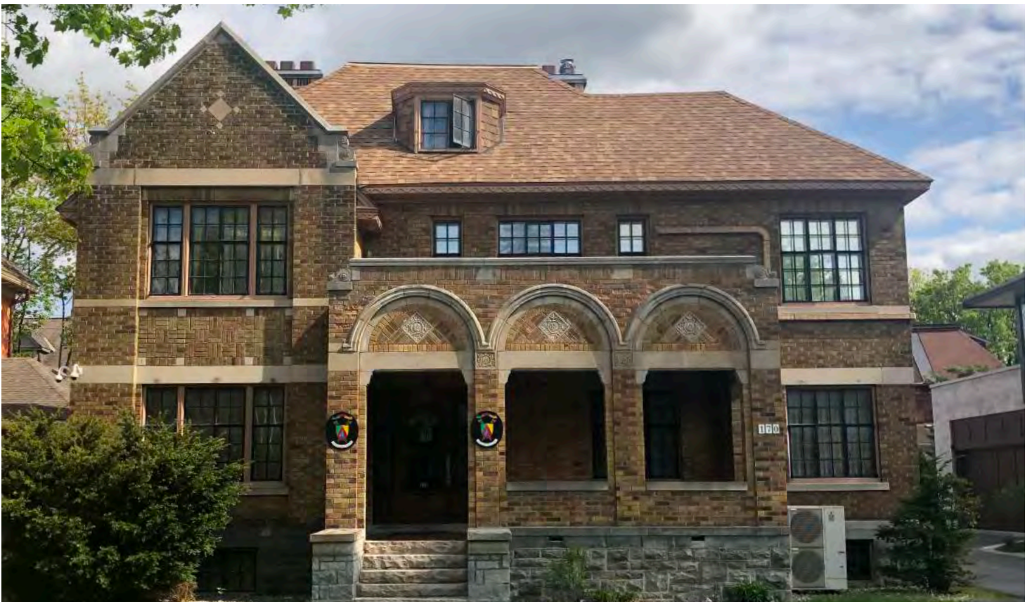
Figure 5: Example of brick cladding with decorative brick detailing
