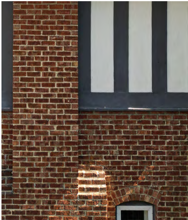
1 EXISTING HALF TIMBERING & BRICK
