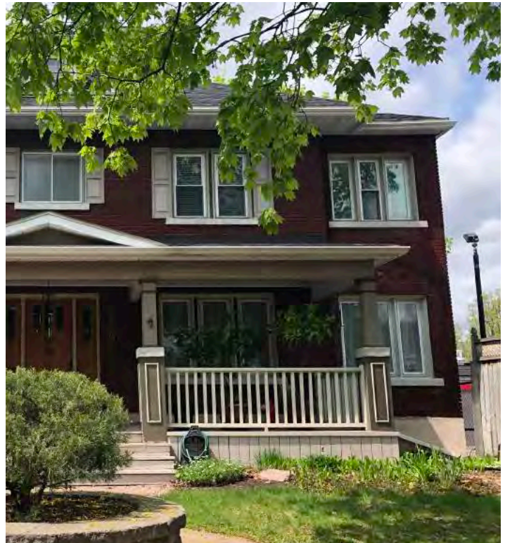
Figure 19: Example of an appropriate addition on right side of house that maintains the brick cladding, alignment of windows, and roof profile.
