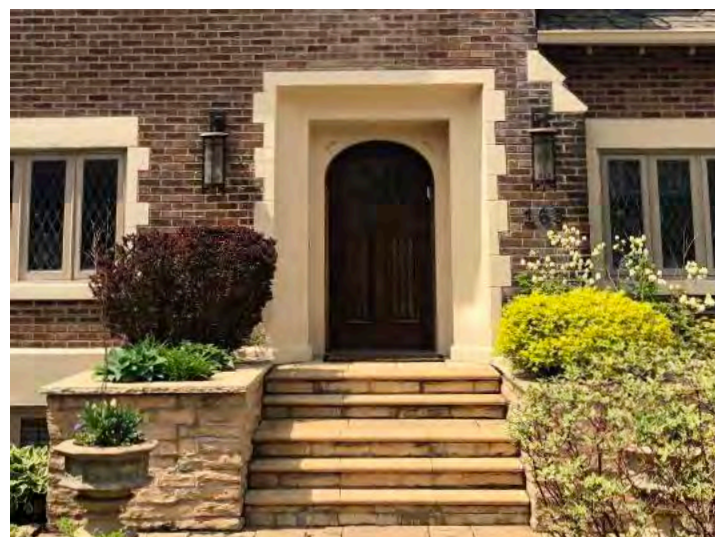
Figure 7: Example of historic elements of door openings
