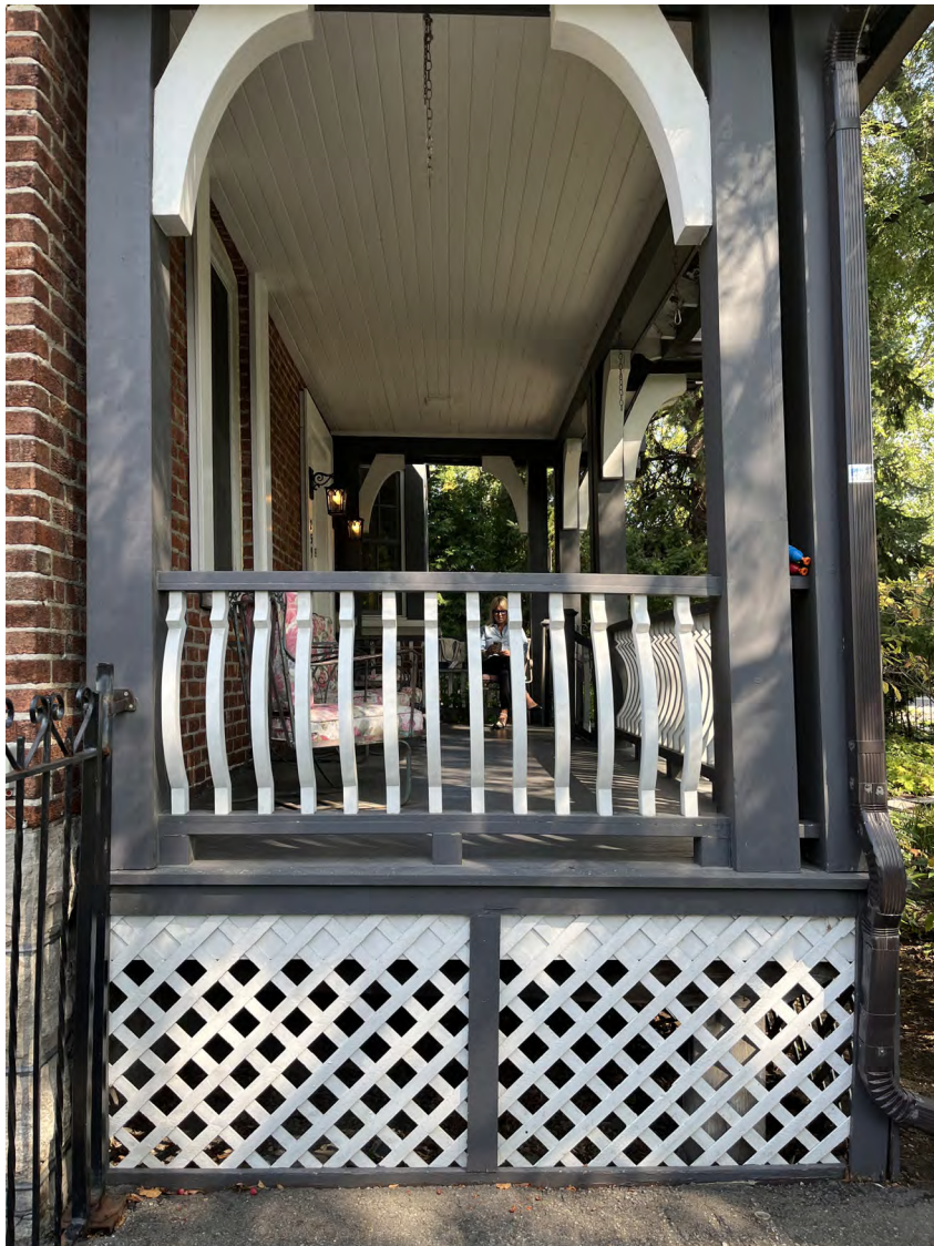
1 EXISTING FRONT PORCH CONDITION
