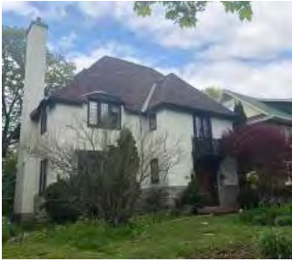
Address: 305 Clemow Construction Date: 1927 Architect: John Bethune Roper
