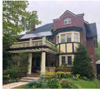
Address: 31 Monkland Construction Date: 1921 Architect: Walter Herbert George
