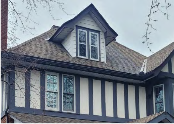
Figure 12 – Existing windows and dormer (RMA+SH, 2024)
