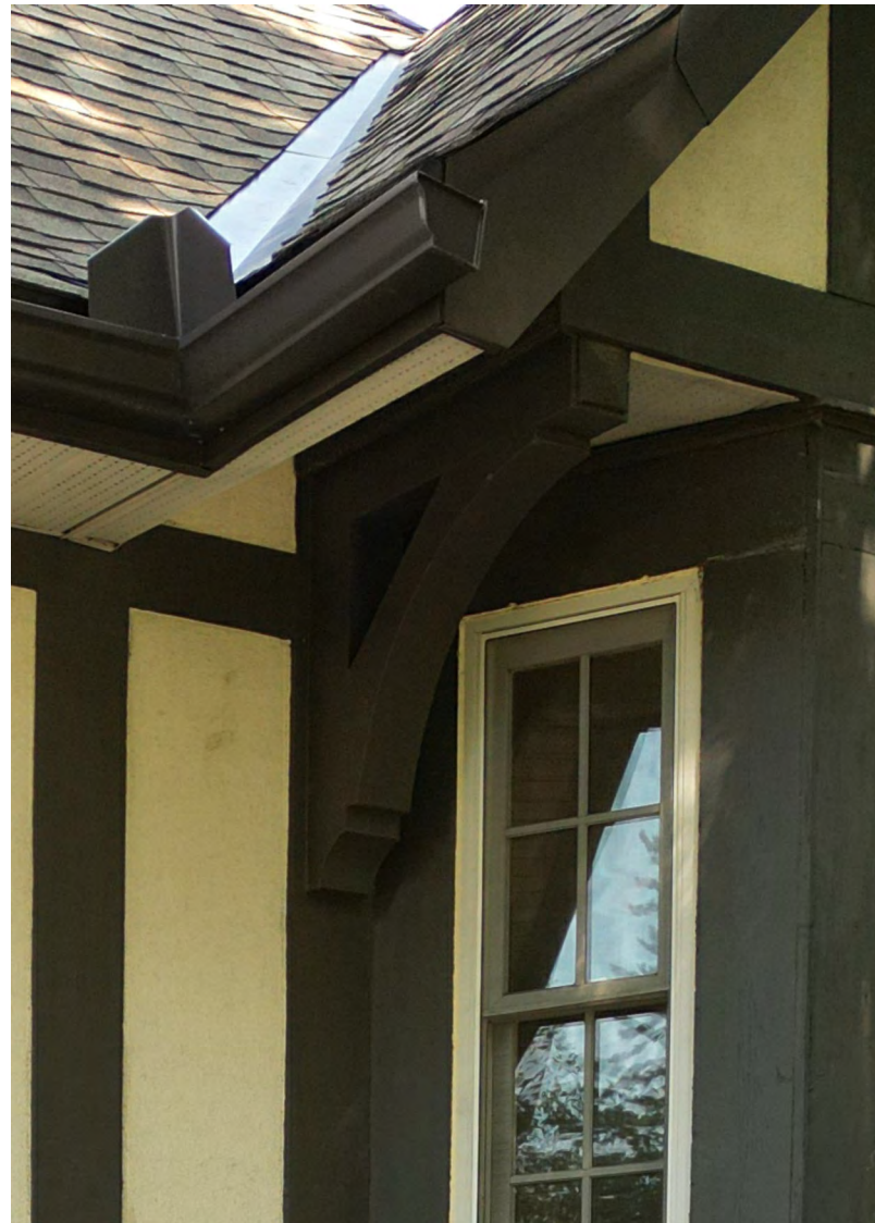
3 EXISTING BAY ORIGINAL BRACKETS - REINSTATE @ PORCH
