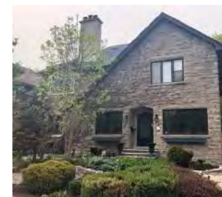
Address: 7 Linden Terrace Construction Date: 1931 Architect: William D. Hopper
