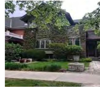
Address: 33 Monkland Construction Date: 1916 Architect: Walter Herbert George
