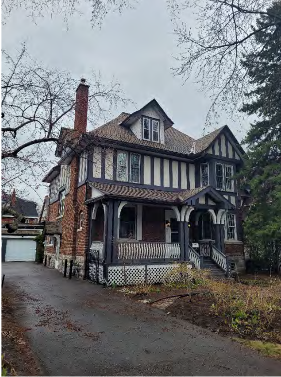
Figure 3 – Current View of 259 Clemow (RMA+SH, 2024)
