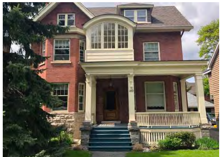
Figure 15: Example of an enclosed upper porch.
