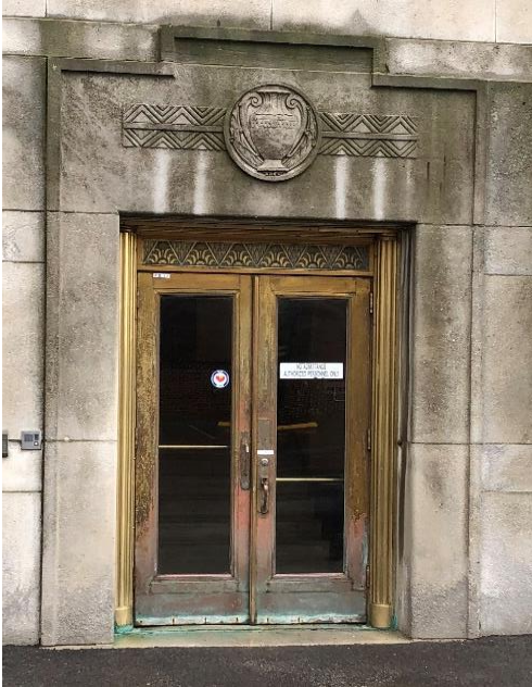
Detail over main entrance
