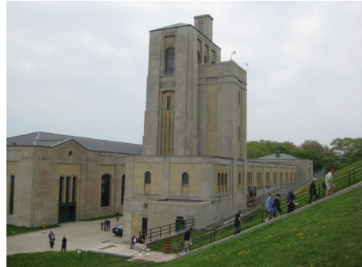
R.C. Harris Water Treatment Plant (Toronto, 1932-1941)
