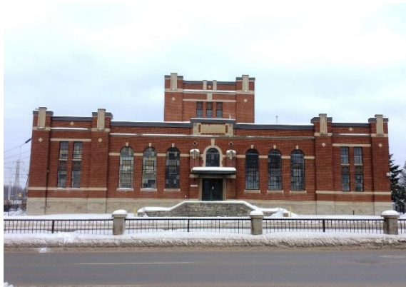
Hydro Sub-Station, 1275 Carling Avenue Ottawa, c. 1929
