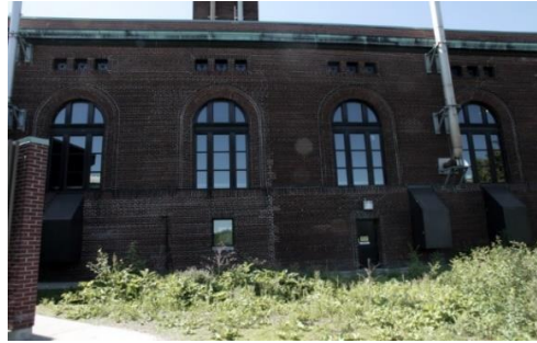
Pumping Station north façade
