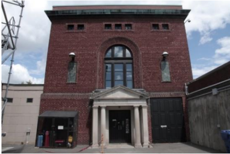
Pumping Station: front elevation
