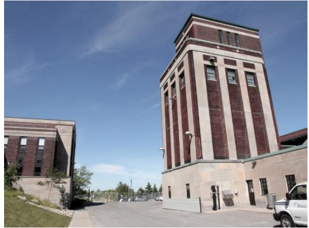
Chemical building tower
