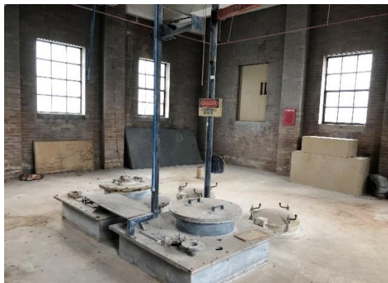
Room with access to container silos
