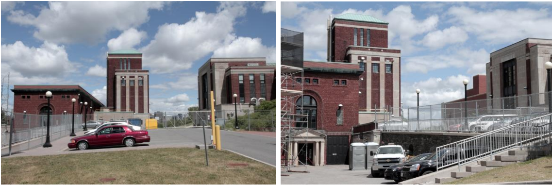
Image: Lemieux Island Water Purification Plant
