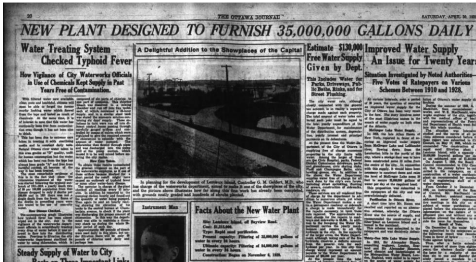
Newspaper coverage of the Opening of Lemieux Island, (April 30, 1932)
