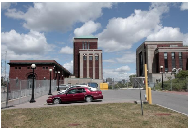
Southern façade of the Chemical Building
