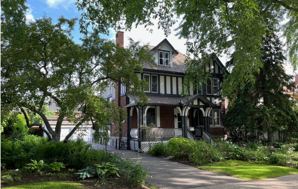
Front (south) and side (west) elevation of 259 Clemow Avenue
