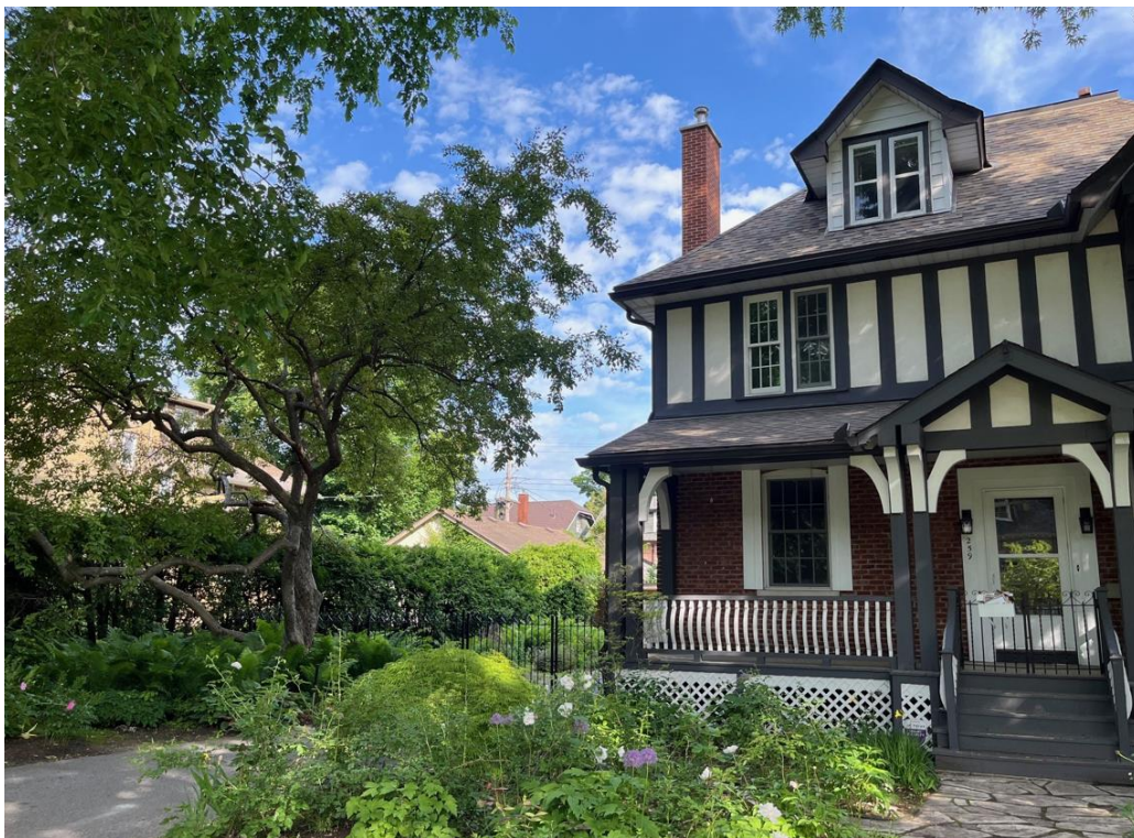
Front elevation (south) of 259 Clemow Avenue
