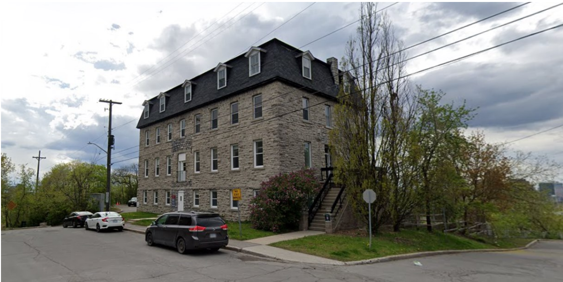
Google Maps (May 2021). South-West view of building.
