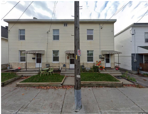
Figure 2-2 The site, north elevation
