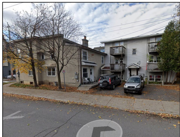
Figure 2-3 The site, north elevation
