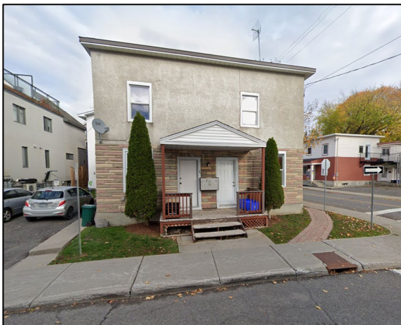
Figure 2-2 The site, east elevation
