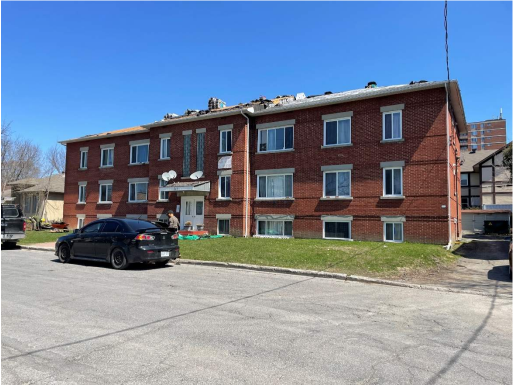
Figure 5. Multi-unit housing across the street to the east, 245 Alfred St.
