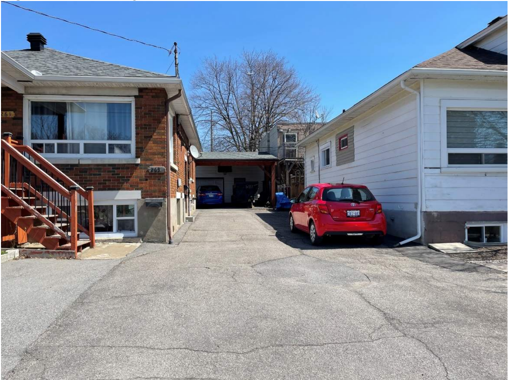
Figure 6. Outbuildings across the street, 259 & 261/263 Alfred St.
