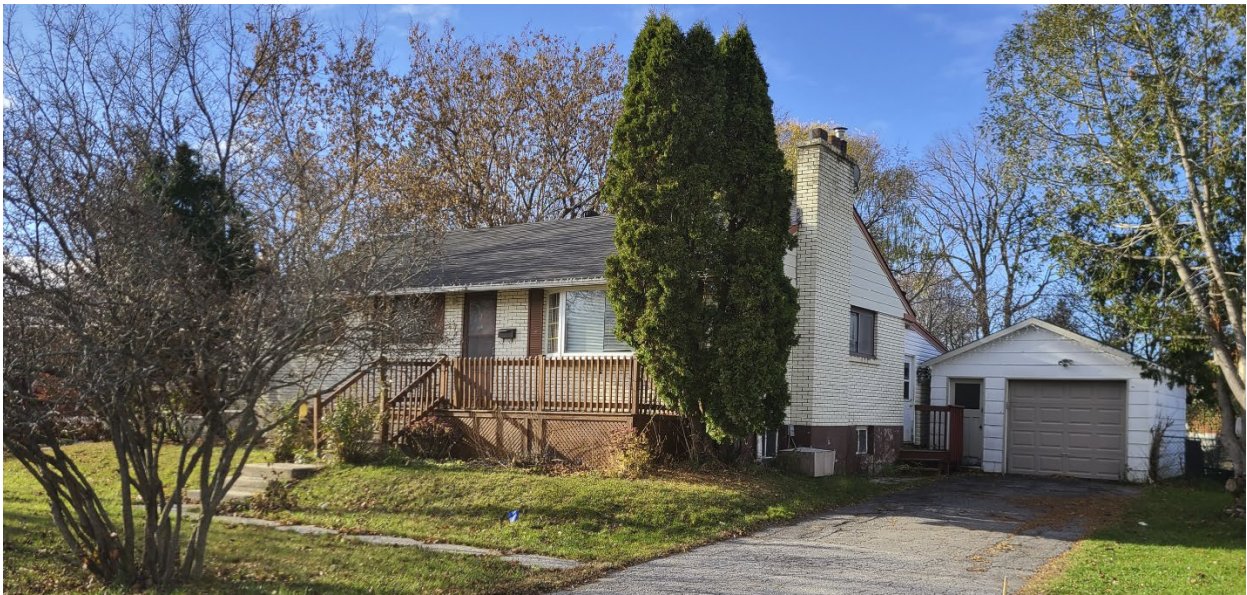
1. Existing Dwelling – North View from Dunham Street
