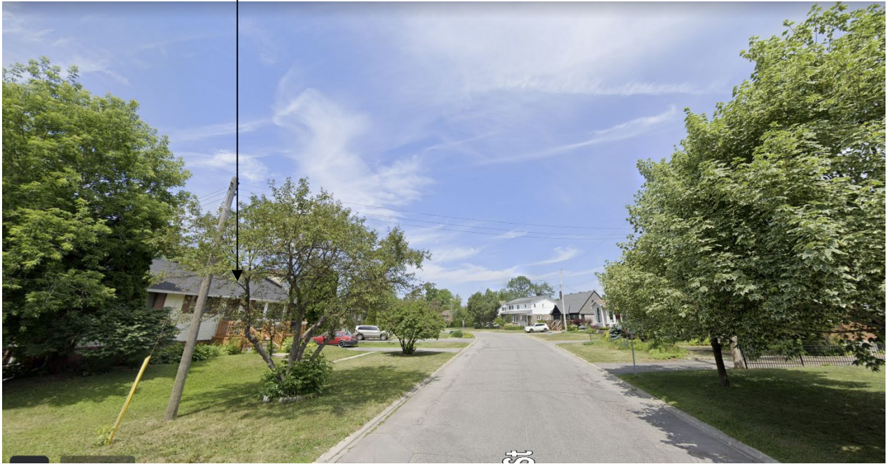
1. Looking north along Dunham Street
