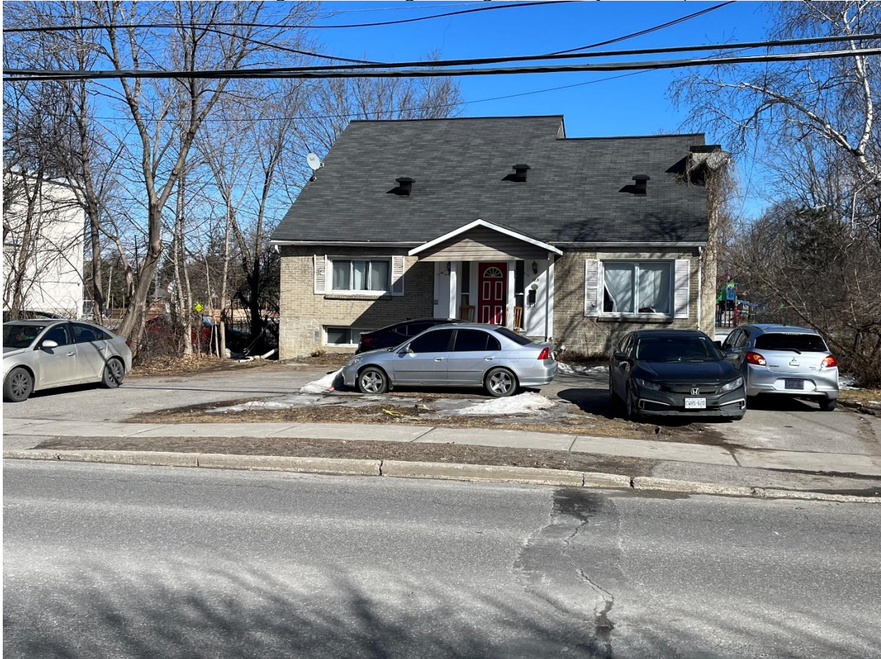
Figure 3: Existing Building on the Subject Site. (Source: Google Maps).
