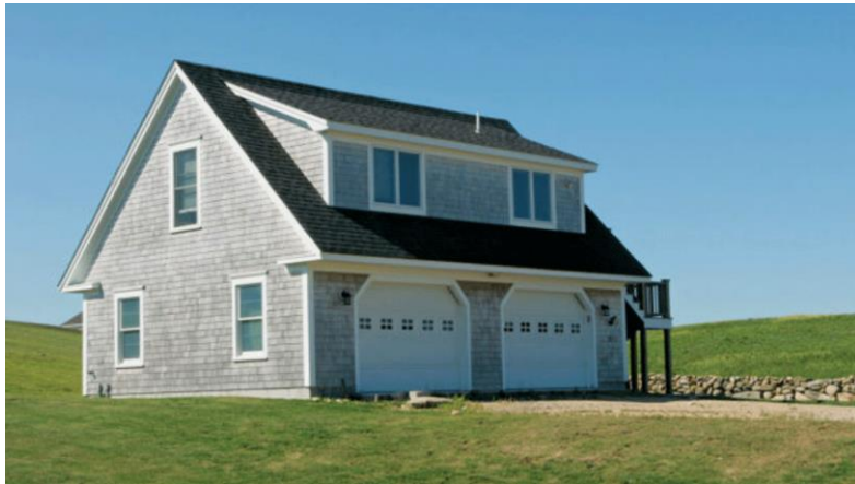
Figure 1. Example photo of a dormer. The dormer is secondary to the main roof line, and does not meet the lower wall.
