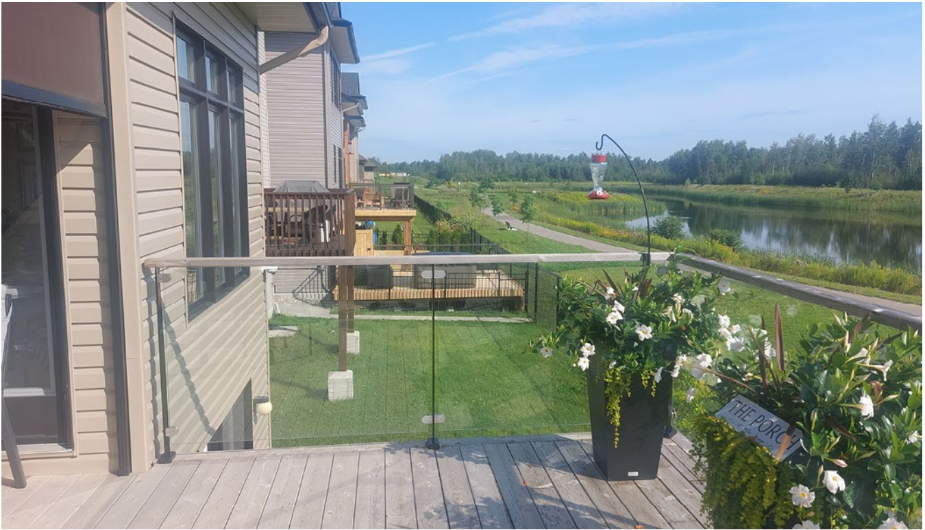
Figure 7: Image taken from the top of deck, identifying similar deck conditions on adjacent properties, looking north.
