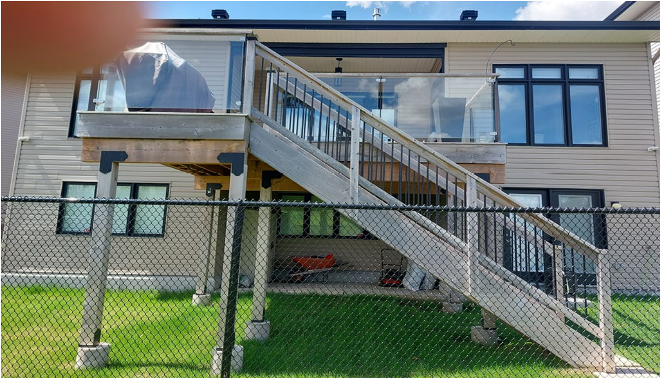
Figure 4: Image of the deck, taken from the area abutting the rear yard of the subject property, looking west.
