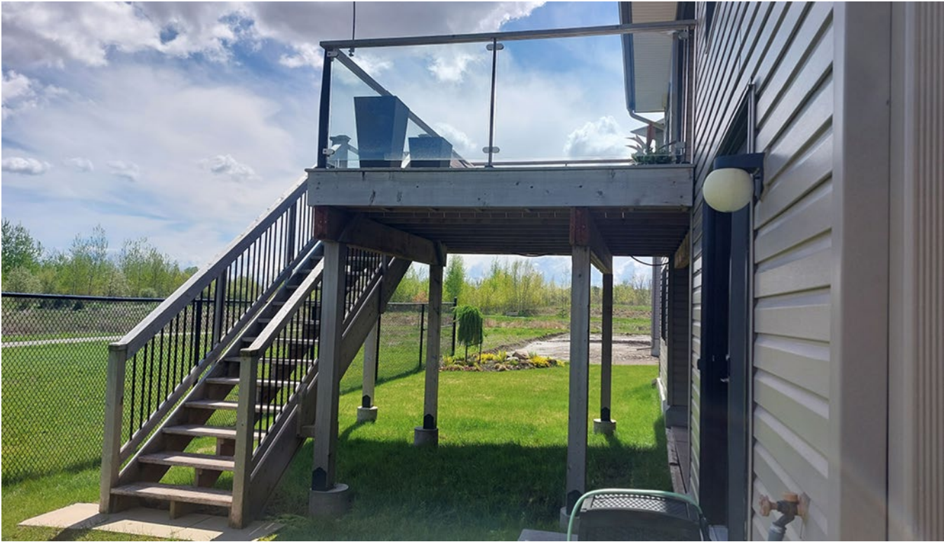
Figure 3: Image of the deck at-grade, looking south.
