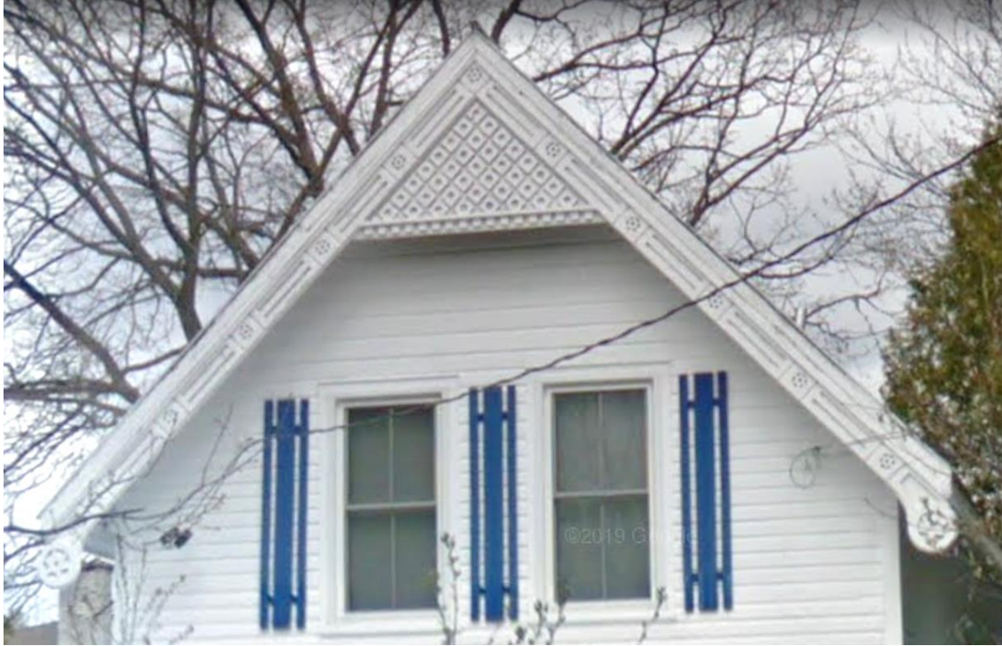
119 Bradford Street, Bargeboard and Gable Apex Panel Detailing, Source: Google Maps, 2016
